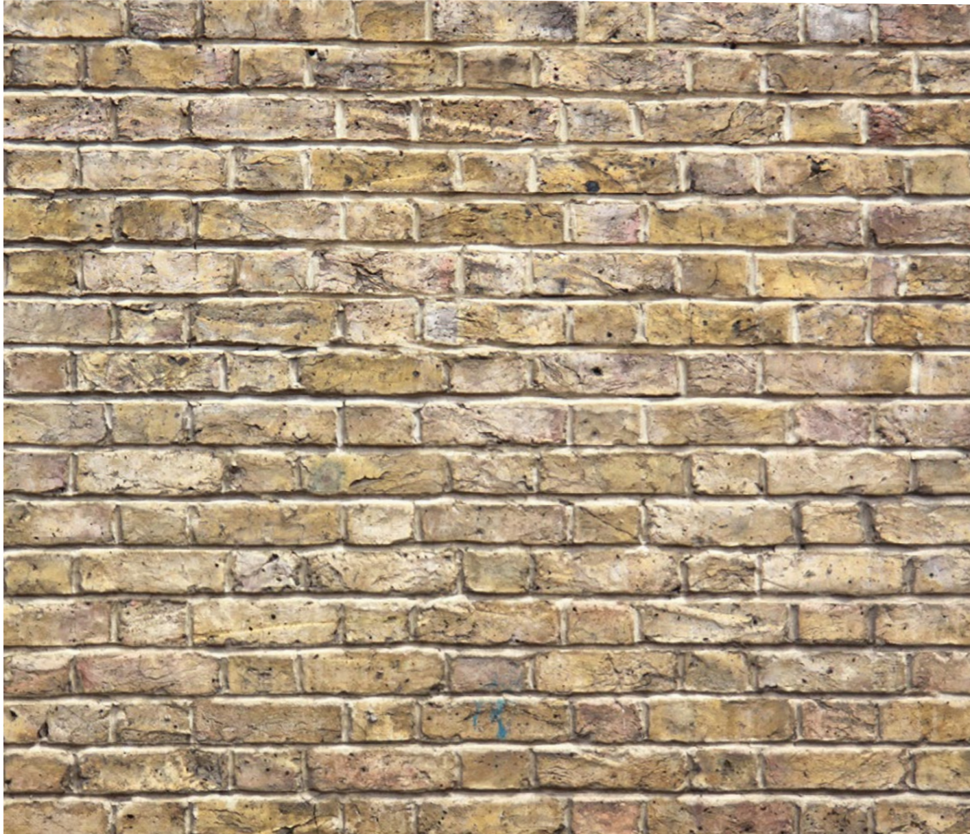
Front boundary and exteriors walls: London stock brick
