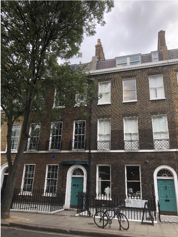
Photograph 1: Front elevation of 48 & 49 Doughty Street
