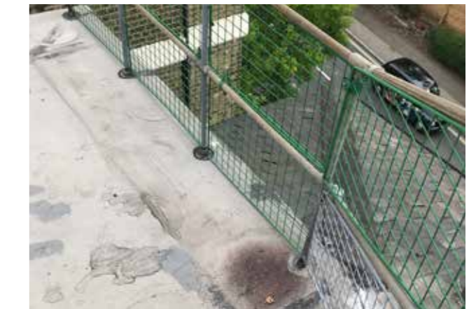
Roof Terrace Balustrade
