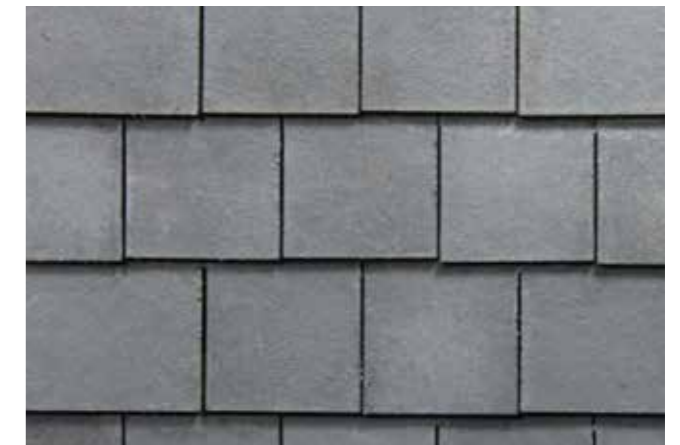
Natural slate tiles to match existing
