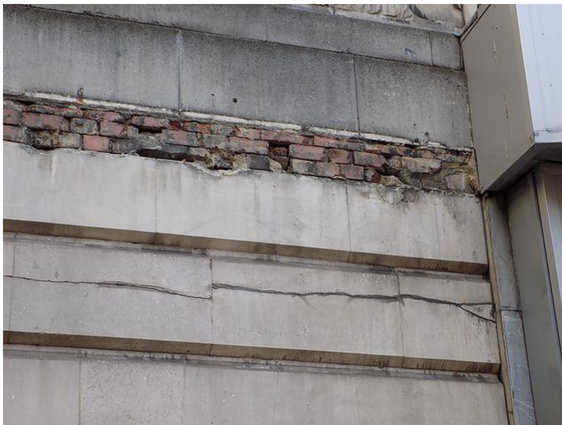
Image 5 – damage to the artificial stone render, with stress cracks from steel frame expansion
