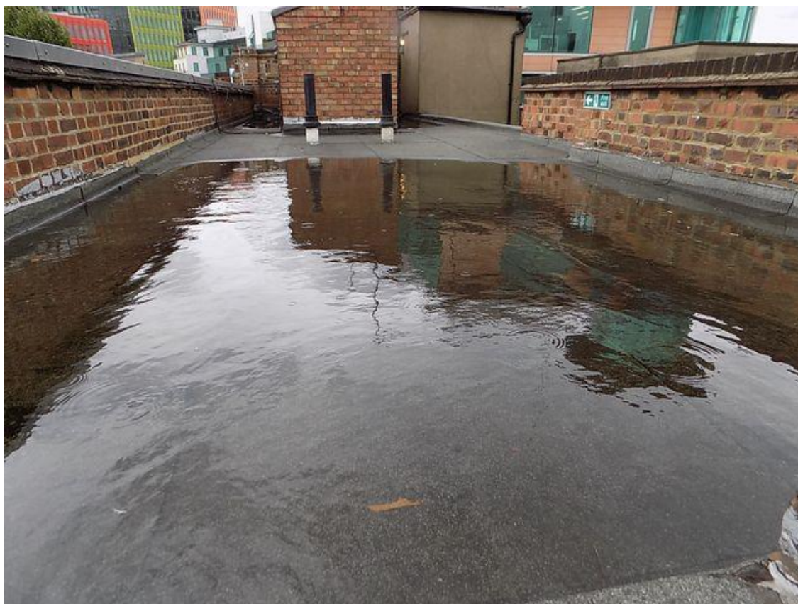
Image 14 – flooded roof surface due to blocked downpipe
