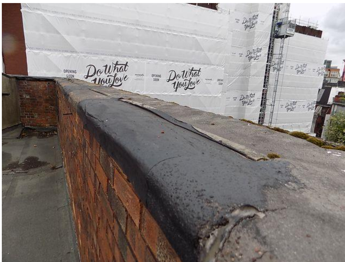
Image 11 – defective asphalt coping
