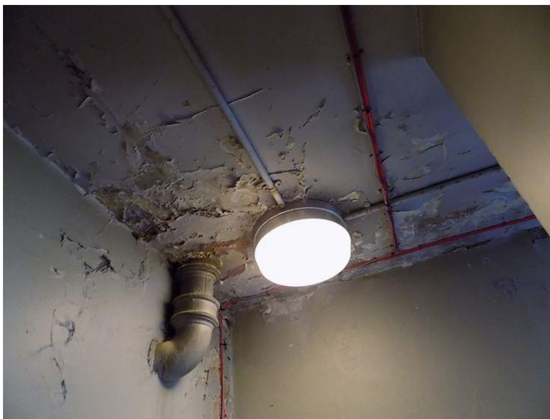
Image 16 – an example of damp penetration through the roof
