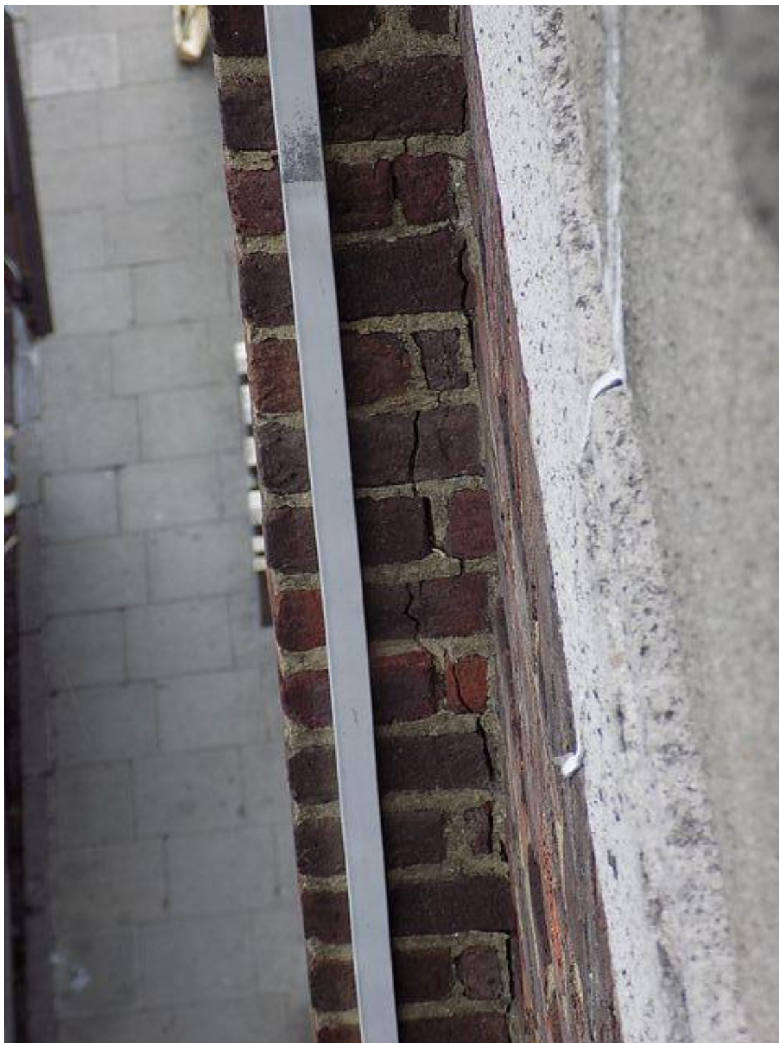
Image 12 – stress cracks in brick skin, presumably due to steel frame corrosion
