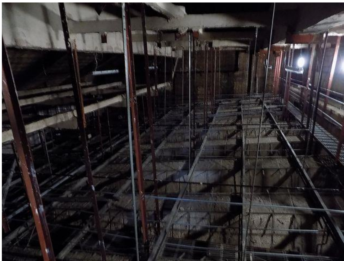
Image 15 – interior of roof, with expanded metal lath ceiling construction supported on a C20 frame
