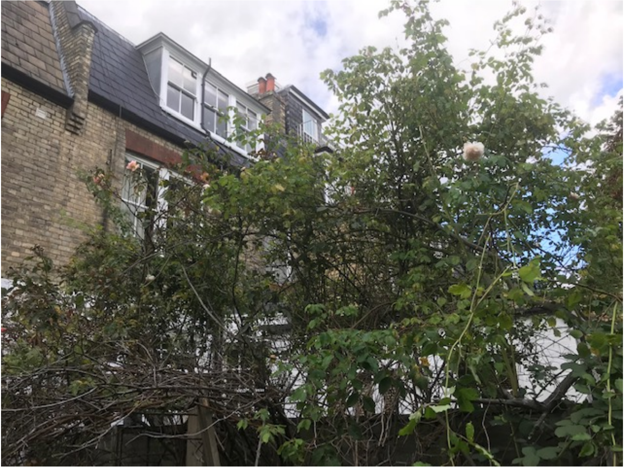
4. Boundary between No. 53 and No. 51 Howitt Road.
