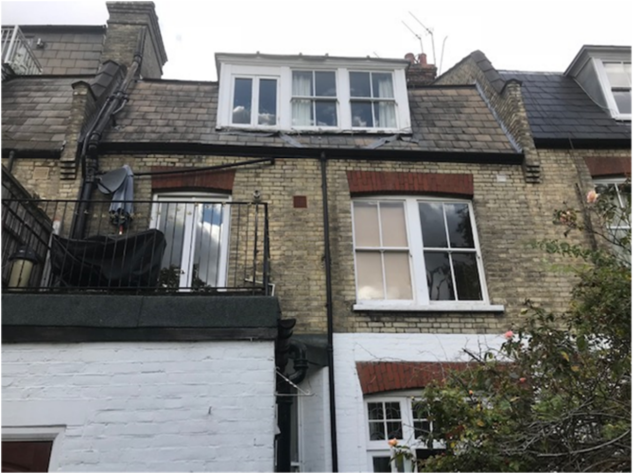
3. Rear elevation (upper floors).
