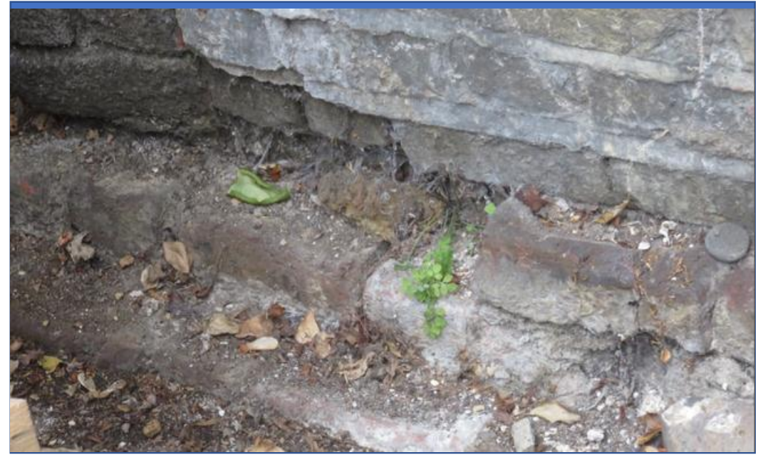
IMG_6118 Base of Party Fence Wall
