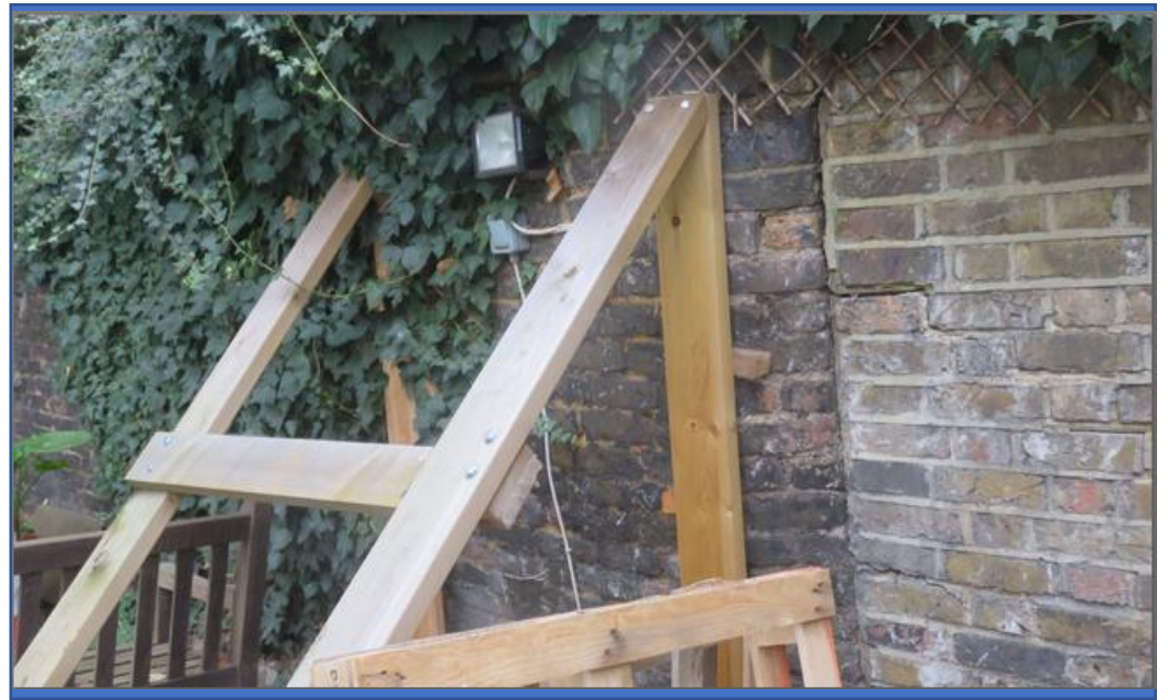
Img_6121 Temporary Support to wall
