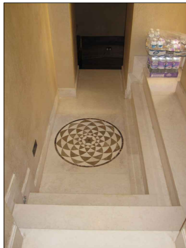
Steps added to a lowered level providing headroom into vaults as approved / existing in 21 Chester Terrace
