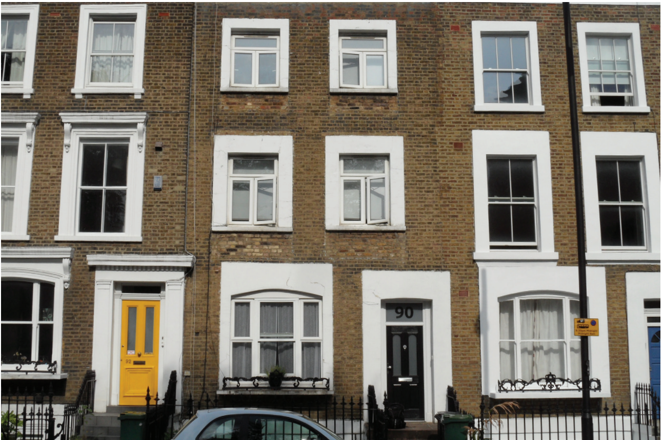
View of front of house (with black door), as existing
