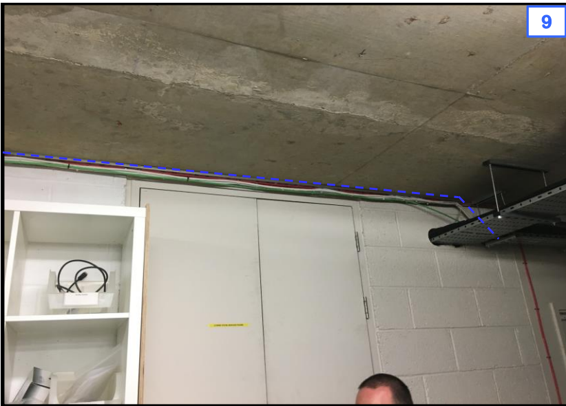
9. 12f cable to follow existing cable route on high level cable tray through basement store and into comms room.
