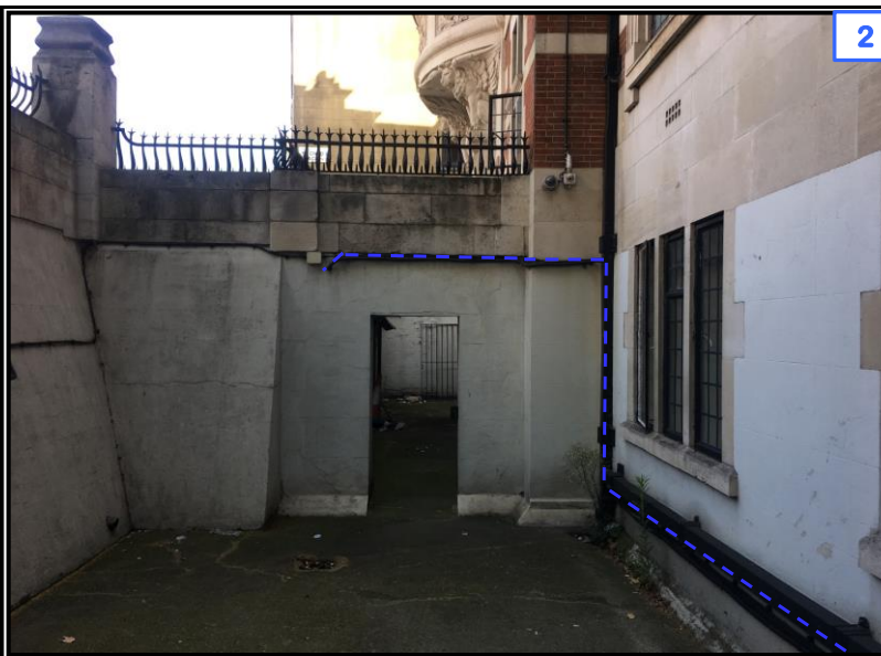
2. 12f cable to follow existing green cable routing through courtyard and towards entrance to basement.
