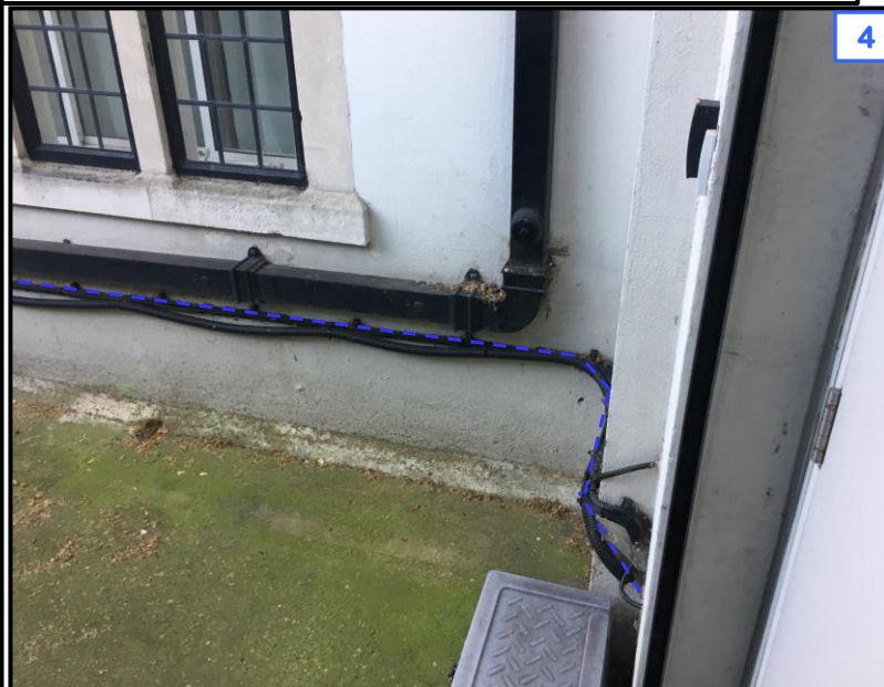
4. 12f cable to follow existing green cable routing through courtyard and towards entrance to basement.
