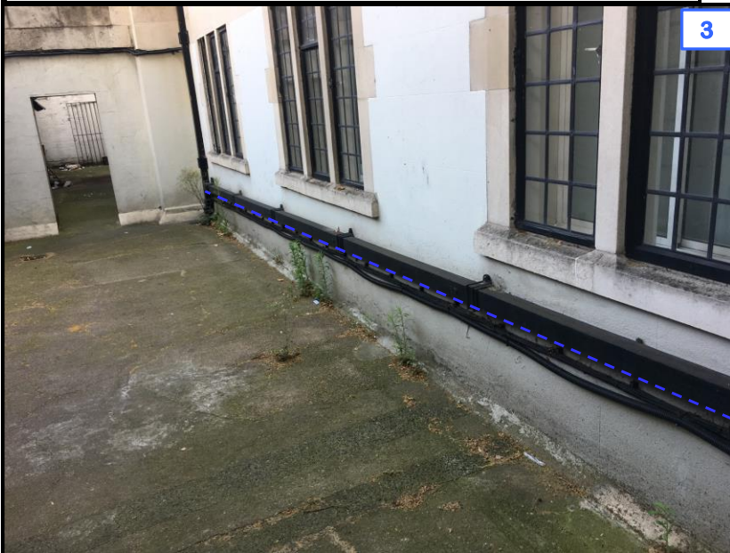
3. 12f cable to follow existing green cable routing through courtyard and towards entrance to basement.
