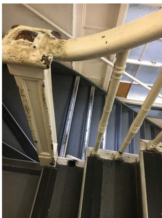
Photograph No.4 - Please refer to the drawing. Missing spindle to be replaced to match the existing. Template to be measured and taken on site and to be replaced to match the existing with pine wood.
