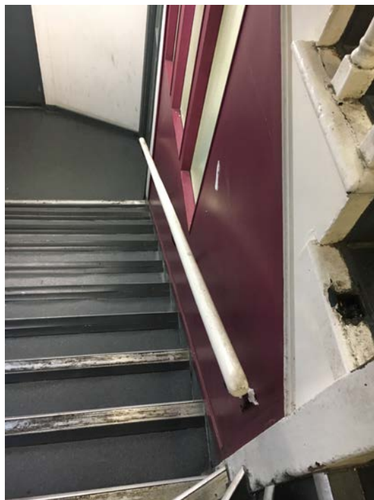
Photograph No.14 – The handrail is to be replaced to match the existing. The handrail is to be removed and a template is to be measured on site. The handrail will be replaced with a pine 40mm mopstick handrail with curves as necessary. The handrail will be painted in Dulux Satinwood Pure Brilliant White Ral:9010
