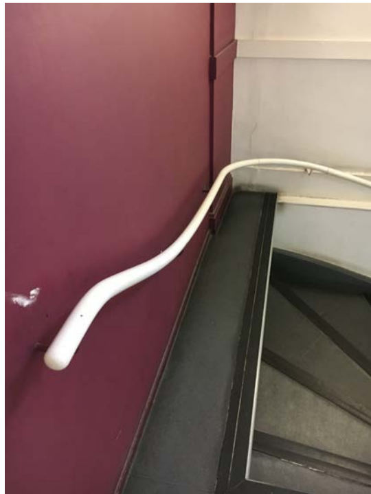
Photograph No.8 – The handrail is to be replaced to match the existing. The handrail is to be removed and a template is to be measured on site. The handrail will be replaced with a pine 40mm mopstick handrail with curves as necessary. The handrail will be painted in Dulux Satinwood Pure Brilliant White Ral:9010
