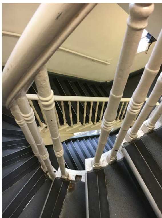
Photograph No. 2 – Please refer to the drawing. Missing spindle to be replaced to match the existing. Template to be measured and taken on site and to be replaced to match the existing with pine wood.
