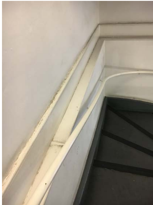
Photograph No.9 – The handrail is to be replaced to match the existing. The handrail is to be removed and a template is to be measured on site. The handrail will be replaced with a pine 40mm mopstick handrail with curves as necessary. The handrail will be painted in Dulux Satinwood Pure Brilliant White Ral:9010
