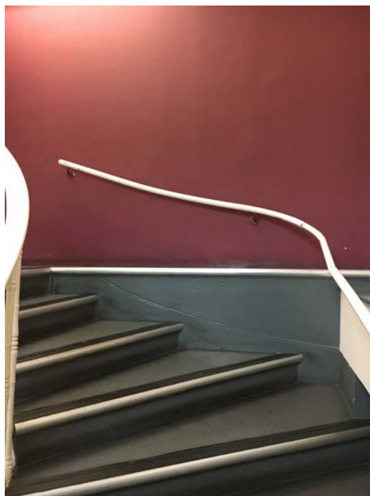
Photograph No.5 – The handrail is to be replaced to match the existing. The handrail is to be removed and a template is to be measured on site. The handrail will be replaced with a pine 40mm mopstick handrail with curves as necessary. The handrail will be painted in Dulux Satinwood Pure Brilliant White Ral:9010
