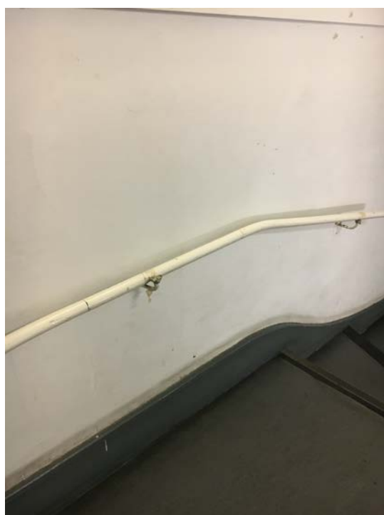
Photograph No.12 – The handrail is to be replaced to match the existing. The handrail is to be removed and a template is to be measured on site. The handrail will be replaced with a pine 40mm mopstick handrail with curves as necessary. The handrail will be painted in Dulux Satinwood Pure Brilliant White Ral:9010
