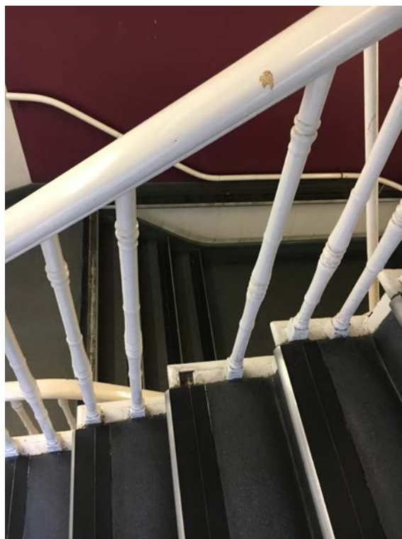
Photograph No.3 - Please refer to the drawing. Missing spindle to be replaced to match the existing. Template to be measured and taken on site and to be replaced to match the existing with pine wood.
