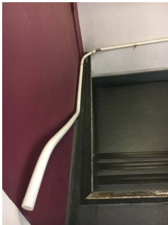
Photograph No.11 – The handrail is to be replaced to match the existing. The handrail is to be removed and a template is to be measured on site. The handrail will be replaced with a pine 40mm mopstick handrail with curves as necessary. The handrail will be painted in Dulux Satinwood Pure Brilliant White Ral:9010
