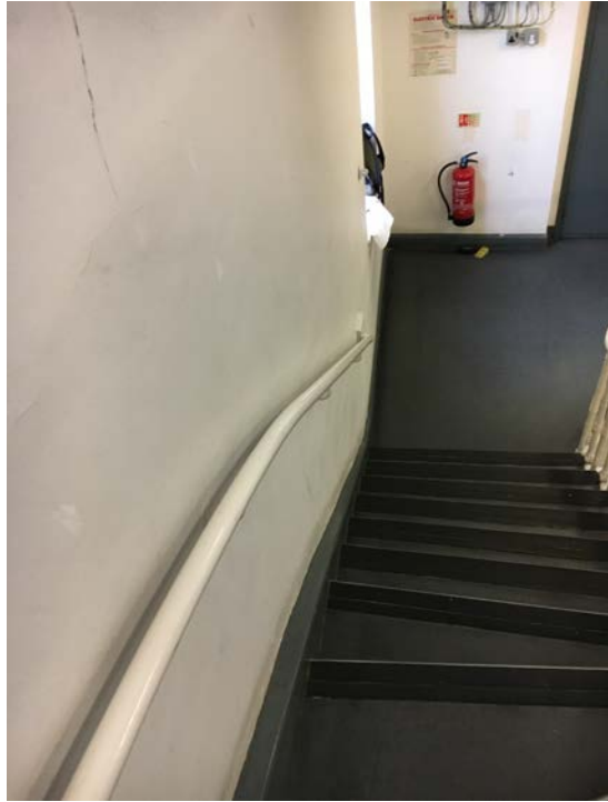
Photograph No.7 – The handrail is to be replaced to match the existing. The handrail is to be removed and a template is to be measured on site. The handrail will be replaced with a pine 40mm mopstick handrail with curves as necessary. The handrail will be painted in Dulux Satinwood Pure Brilliant White Ral:9010
