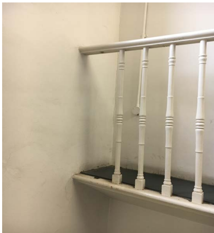
Photograph No.1 – Please refer to the drawing. Missing spindle to be replaced to match the existing. Template to be measured and taken on site and the be replaced to match the existing with pine wood.
