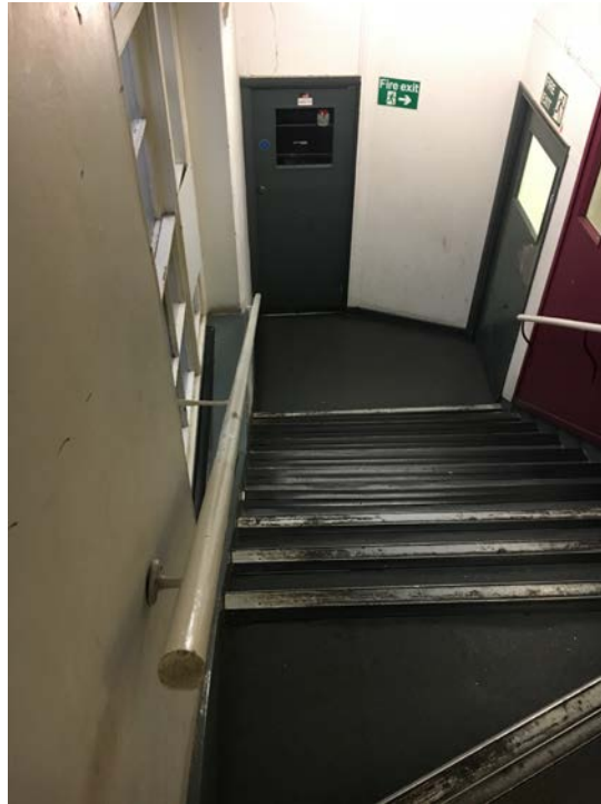
Photograph No.13 – The handrail is to be replaced to match the existing. The handrail is to be removed and a template is to be measured on site. The handrail will be replaced with a pine 40mm mopstick handrail with curves as necessary. The handrail will be painted in Dulux Satinwood Pure Brilliant White Ral:9010
