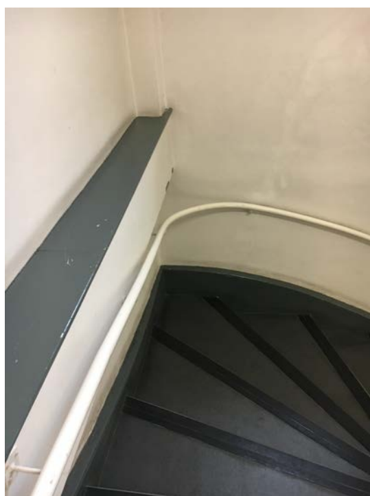
Photograph No.6 – The handrail is to be replaced to match the existing. The handrail is to be removed and a template is to be measured on site. The handrail will be replaced with a pine 40mm mopstick handrail with curves as necessary. The handrail will be painted in Dulux Satinwood Pure Brilliant White Ral:9010
