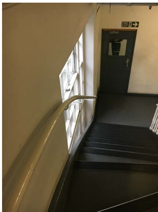
Photograph No.10 – The handrail is to be replaced to match the existing. The handrail is to be removed and a template is to be measured on site. The handrail will be replaced with a pine 40mm mopstick handrail with curves as necessary. The handrail will be painted in Dulux Satinwood Pure Brilliant White Ral:9010
