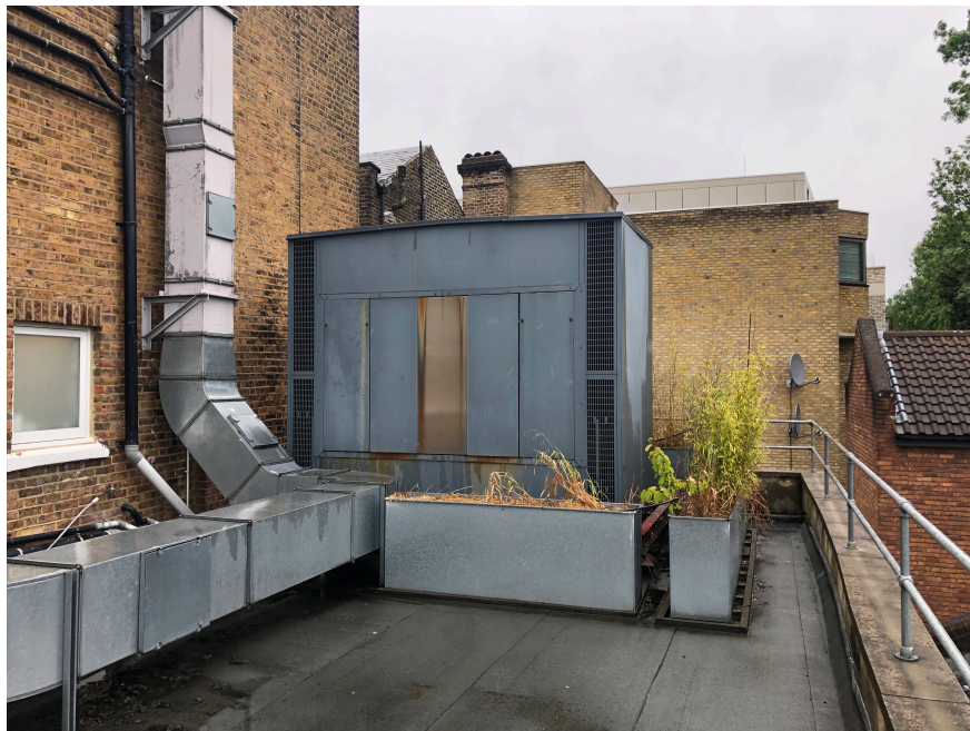
Photograph of the rear facade
