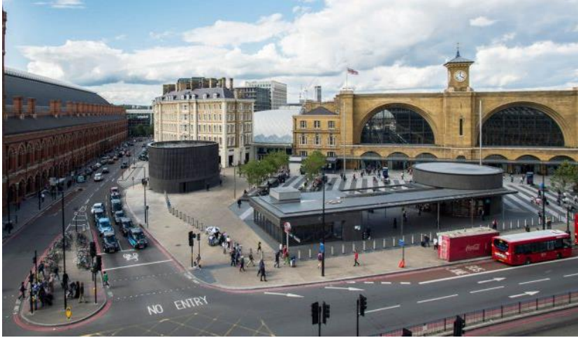
View over Kings Cross and St Pancras Station from the site
