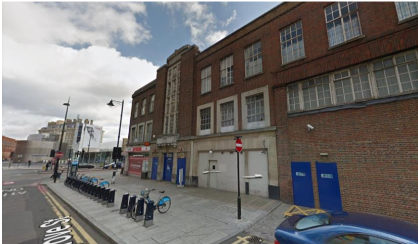
Access Storage at Belgrave House, opposite the site
