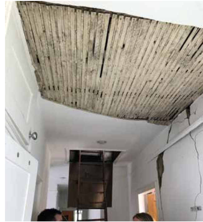
Internal photographs showing extend of cracking
