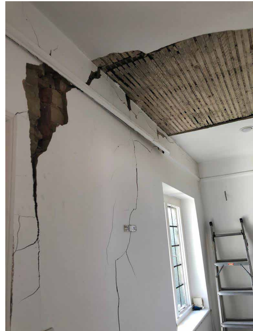
Internal photographs showing extend of cracking, subsidence and ceiling condition
