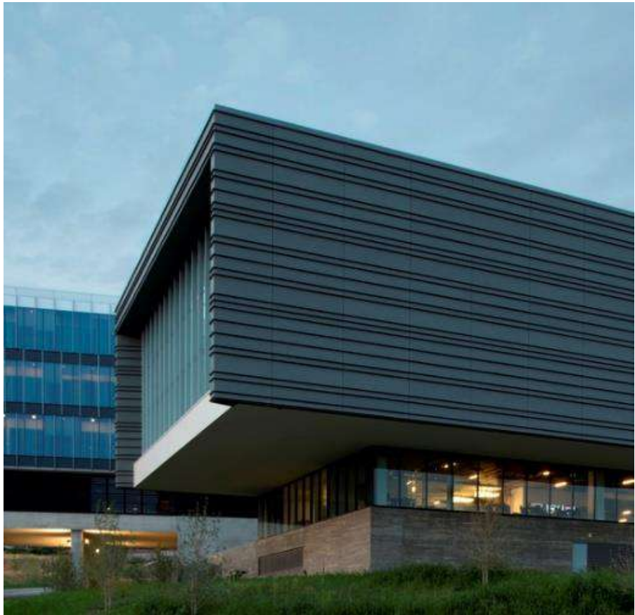
PPC aluminium oxidised coating rainscreen cladding
