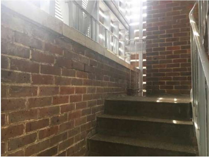
Non-compliant existing concrete risers
