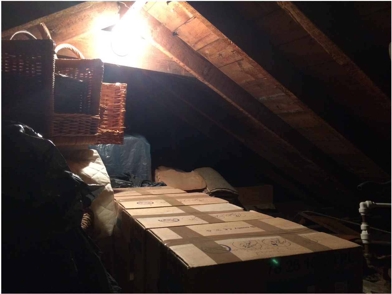
general view of roof space
