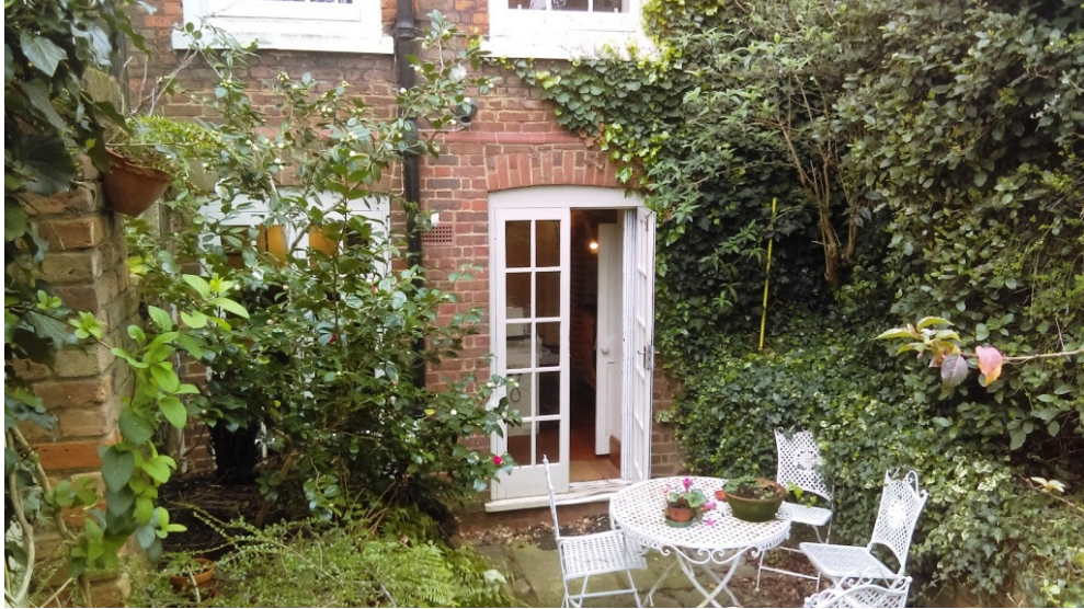
1.1 View of lower ground floor rear elevation. Proposed boiler flue to be located to right hand side of French doors.
