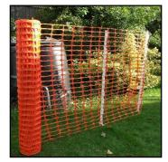
and shall define the working space for the foot operatives, prevent straying into other root protection areas and minimise landscape disturbance. 100mm diameter tops fencing stakes placed at 4m intervals shall be driven at least 0.6m into ground. Plastic barrier material (see left) 1m in height shall be stapled to the stakes so as to form a continuous barrier.
