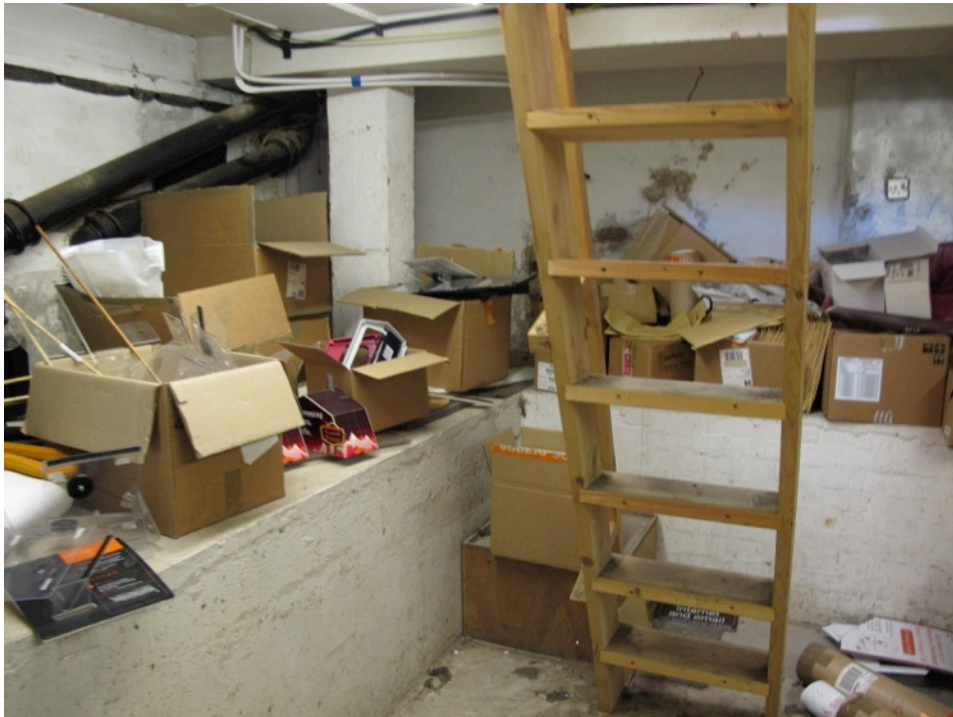
Existing hatch access to basement storage (photo showing previous use)
