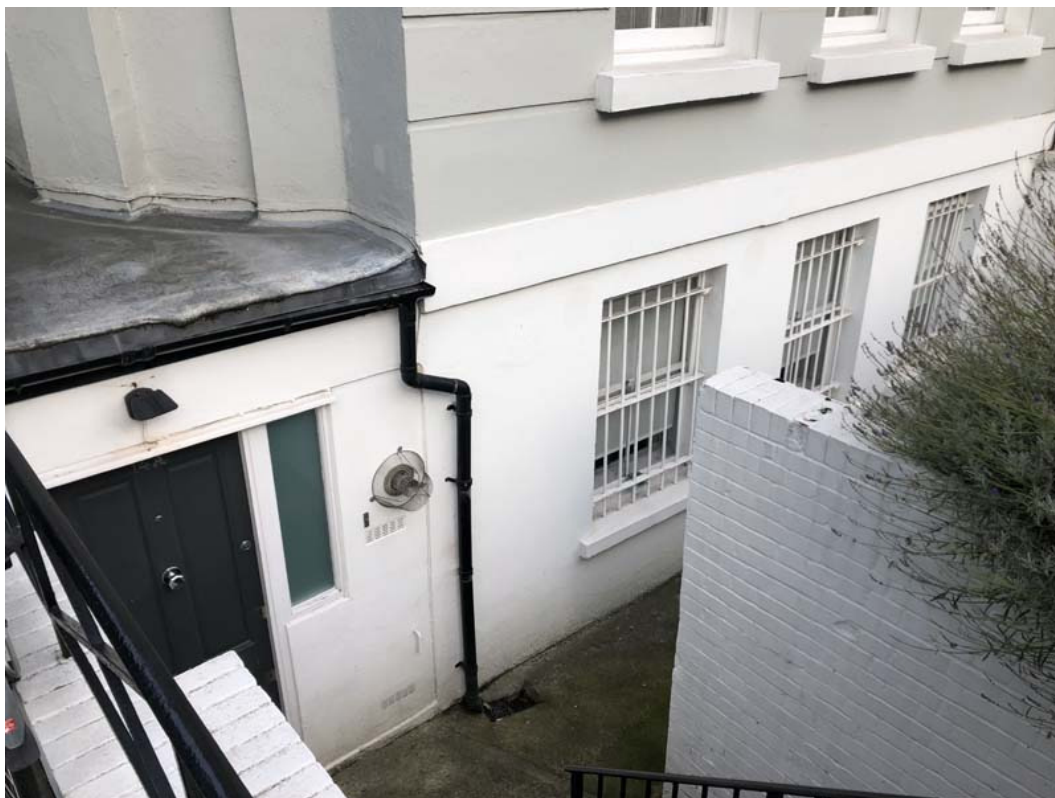
View of basement front.
