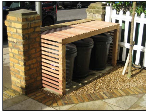
Example of cycle store with pervious base e.g. Duobloc
