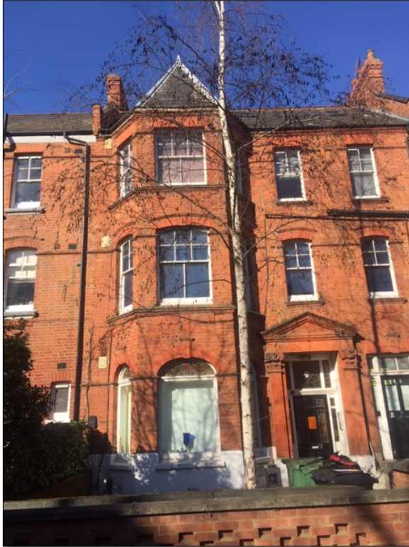
Fig 1: View of 28 Canfield Gardens with T1 in the foreground
