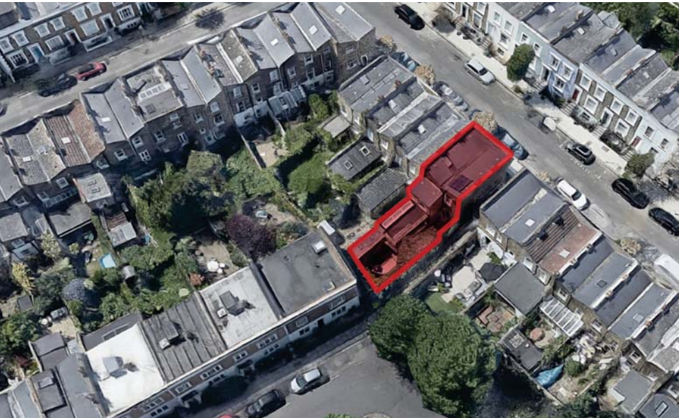
Aerial view showing no. 9 Inkerman Road
