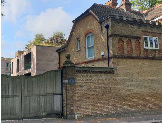
Figure 6: Street View- Existing
