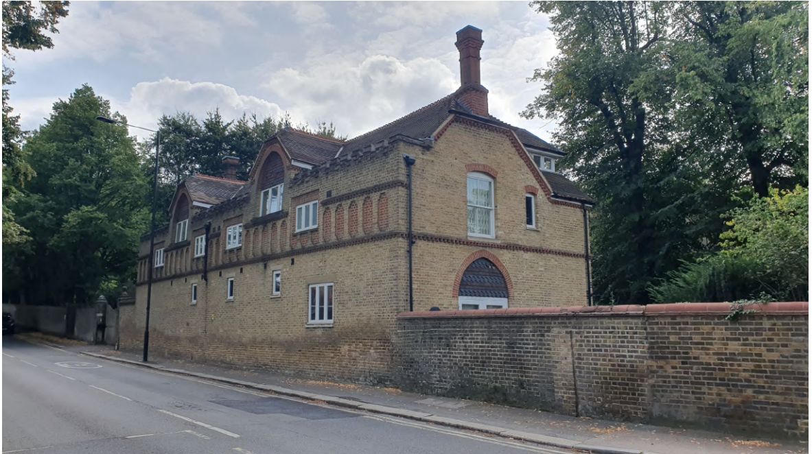
Figure 3: Front elevation of the Coach House from Hampstead Lane
