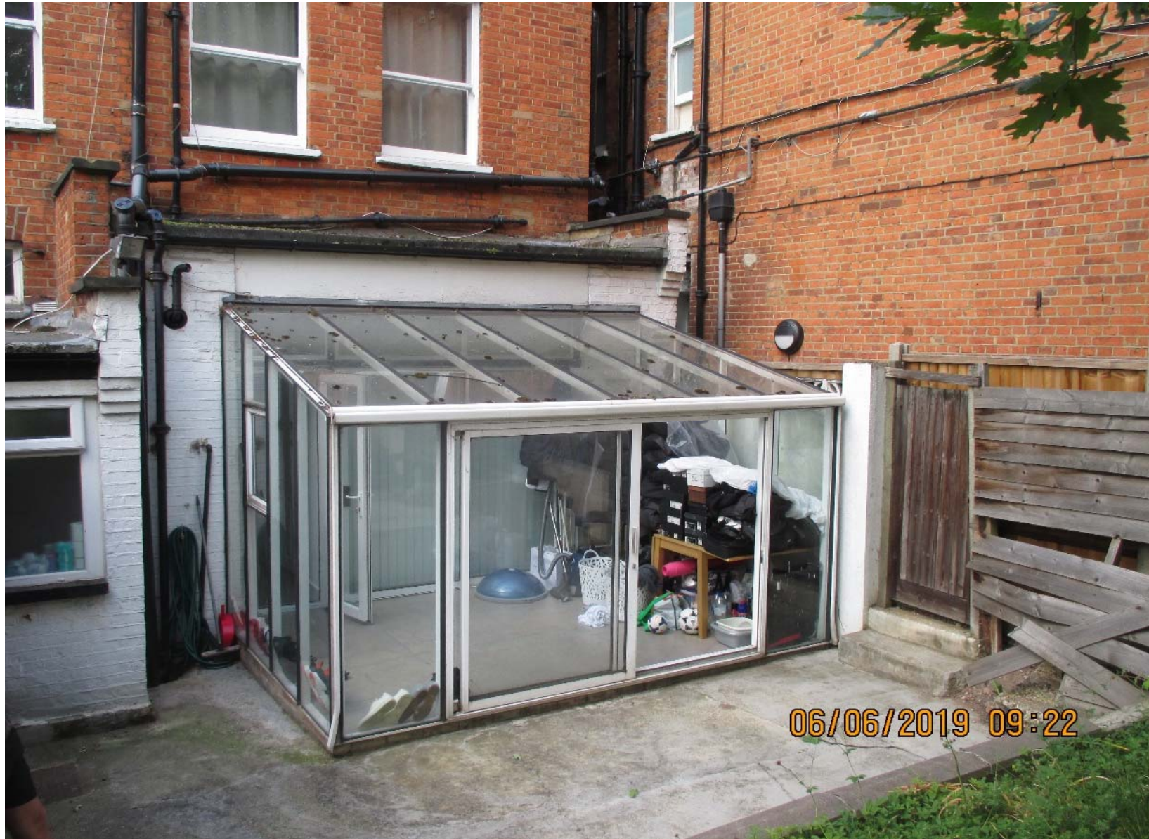
Existing conservatory to be demolished
