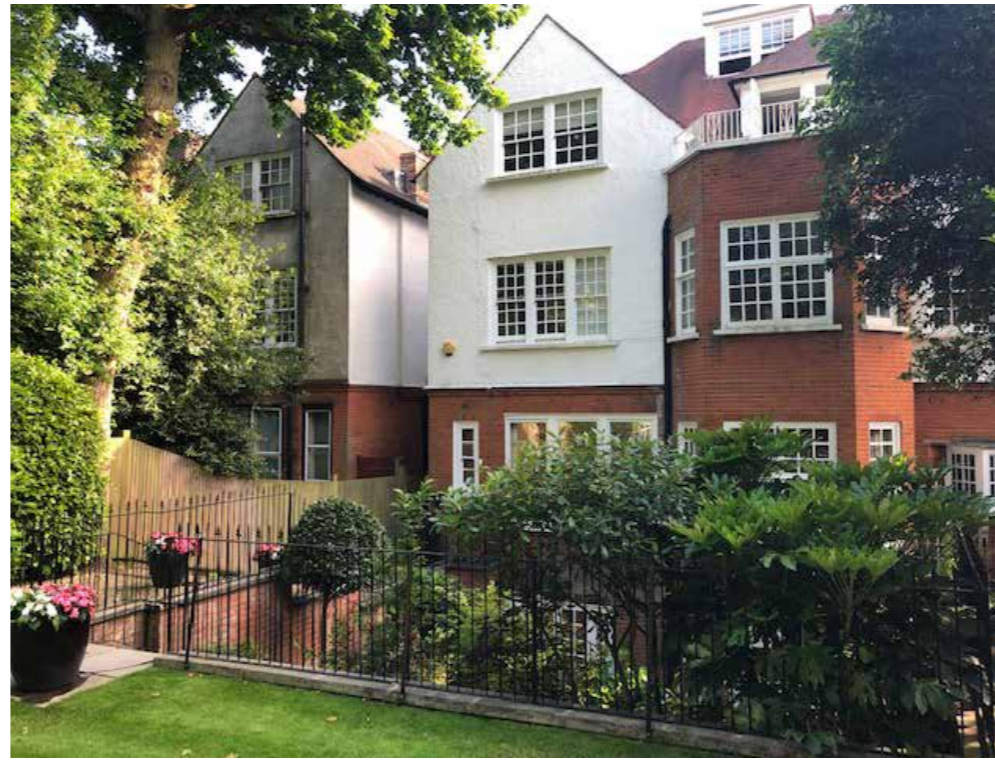
rear elevation bracknell gardens
