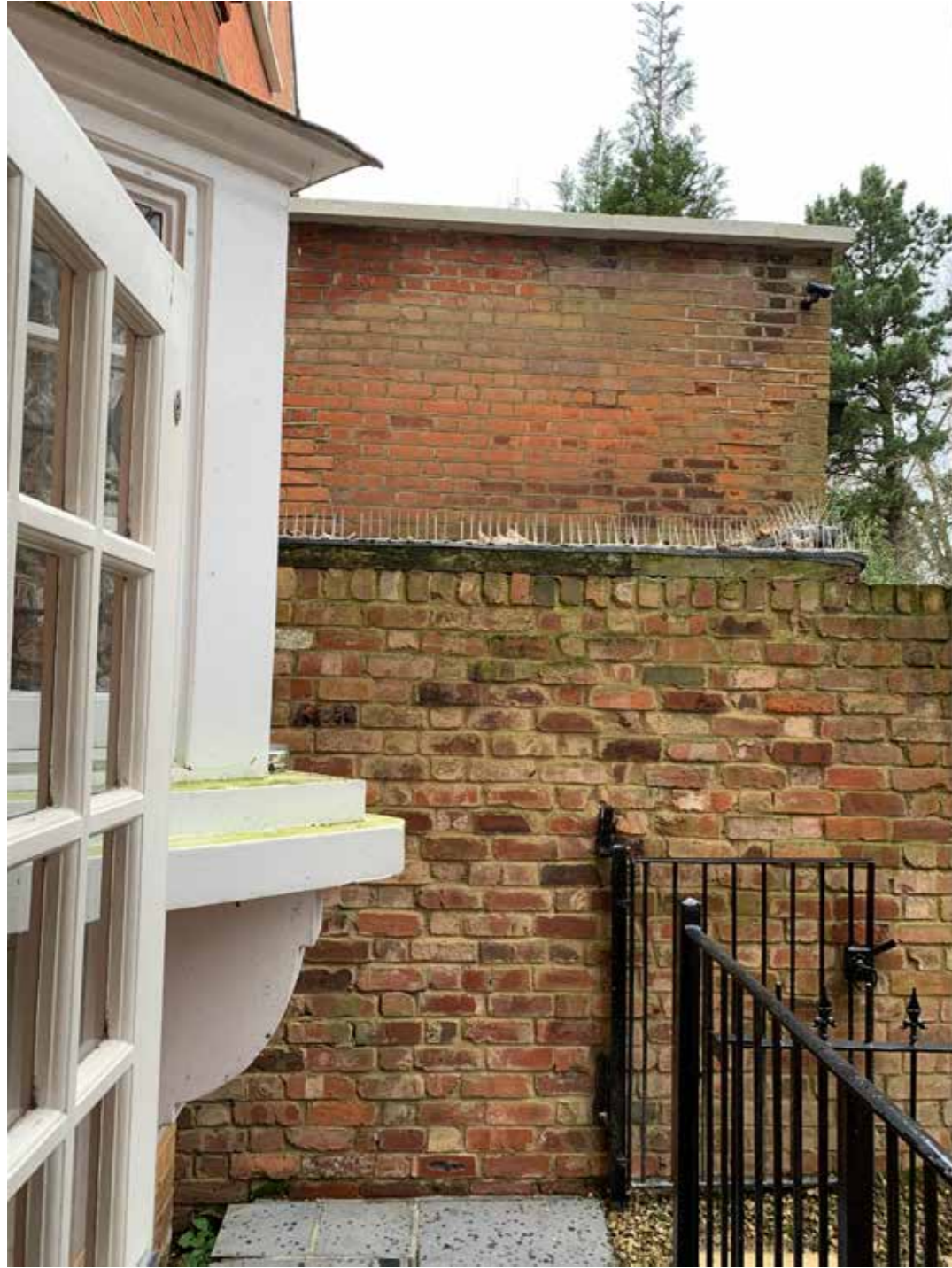
ground floor extension to no.12 bracknell gardens
