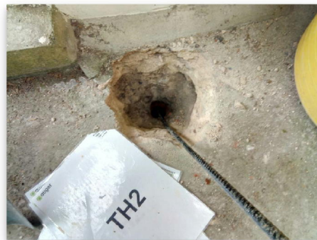
Fig 2.2: Trial Hole 2 Footing
