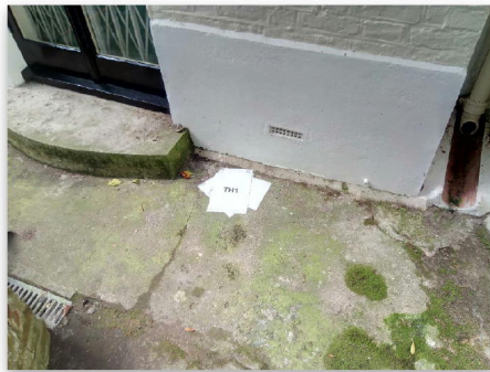
Fig 1.1: Trial Hole 1 Location
