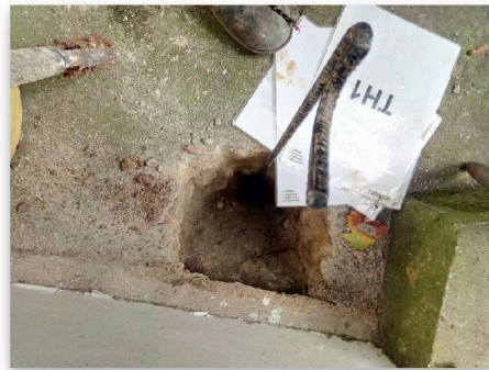
Fig 1.2: Trial Hole 1 Footing
