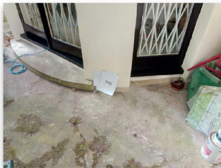
Fig 2.1: Trial Hole 2 Location
