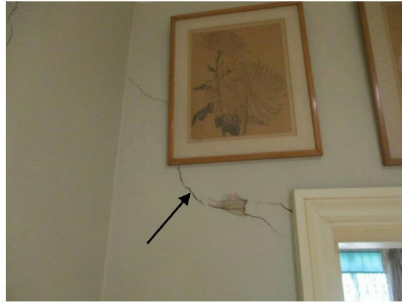
Cracking in basement flat hallway
