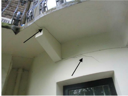
Cracking to rear bay
