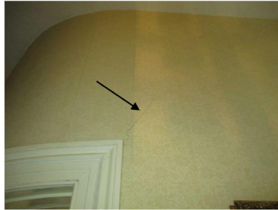
Cracking in flat 1 hallway
