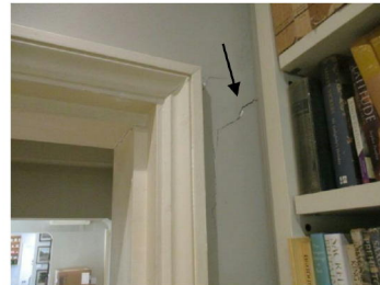
Cracking in basement flat rear bedroom
