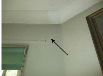
Cracking to bay in basement flat lounge
