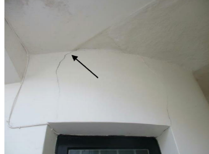
Cracking to rear bay
