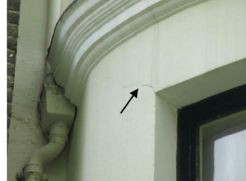
Cracking to rear bay
