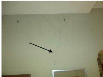
Cracking in basement flat hallway
