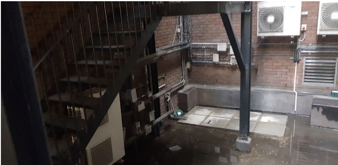
Area at Base of Lightwell
