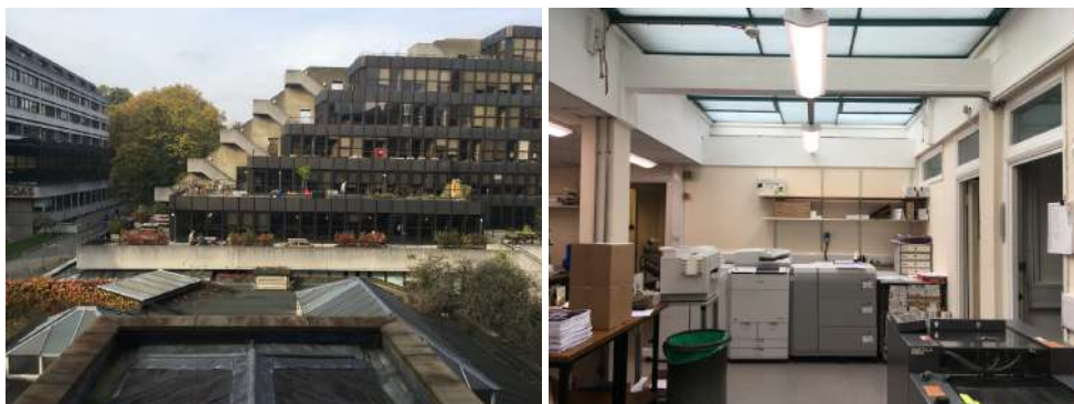
Figs. 08 & 09 - Existing roof layout with lanterns and internal secondary glazing
