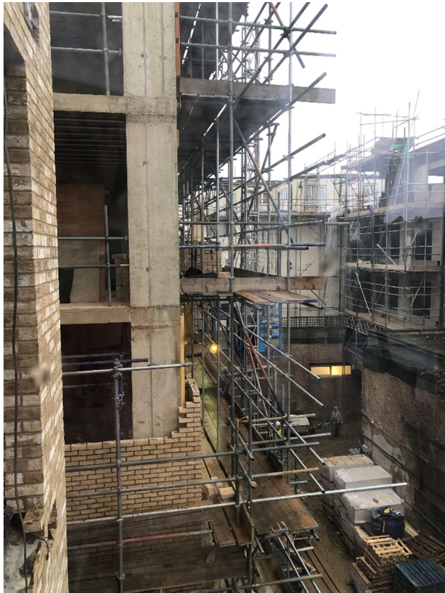
Figure 7 - Flat 312 balcony view, brick flank wall under construction
