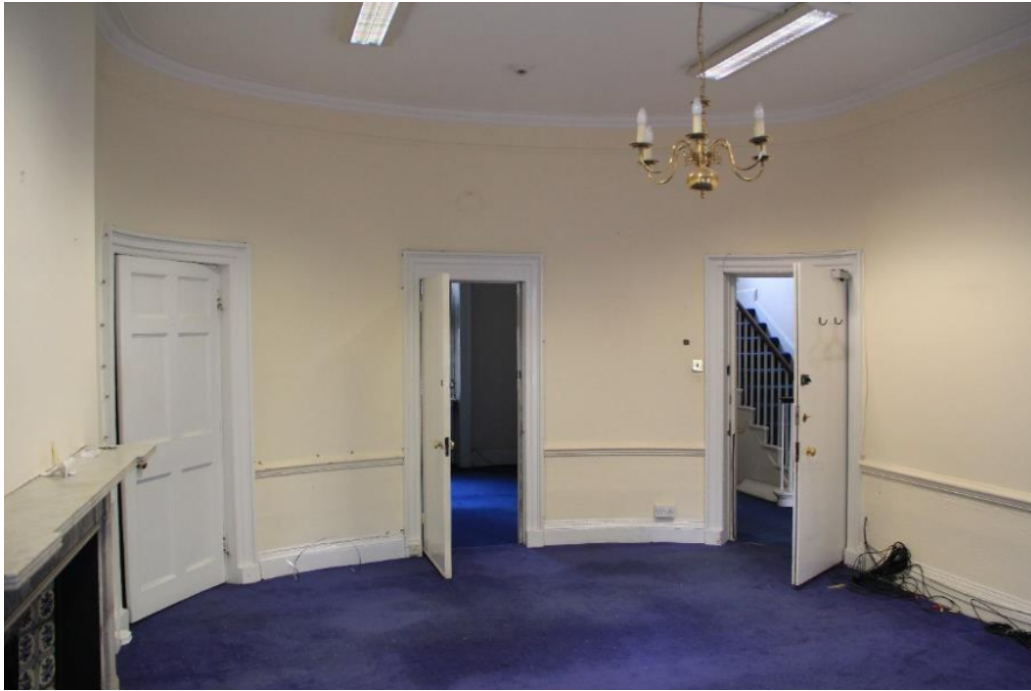
7. Existing curved wall in front room at ground floor level.
