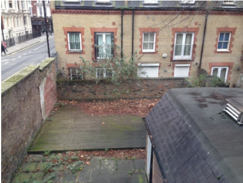
5. Existing rear garden and rear extension
