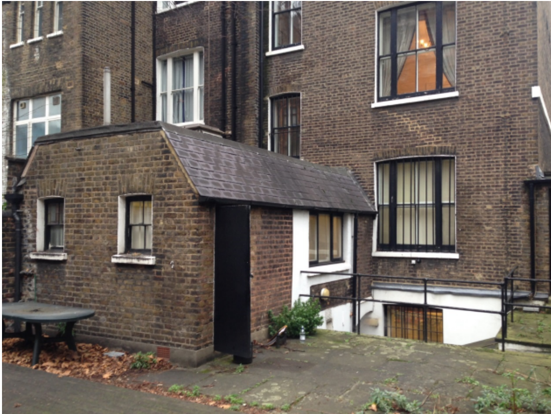
1. Rear elevation, existing rear extension and rear lighwell.
