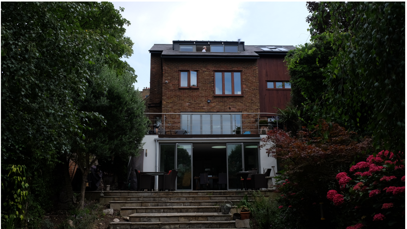
Photo 2 – west elevation taken from bottom of garden.
