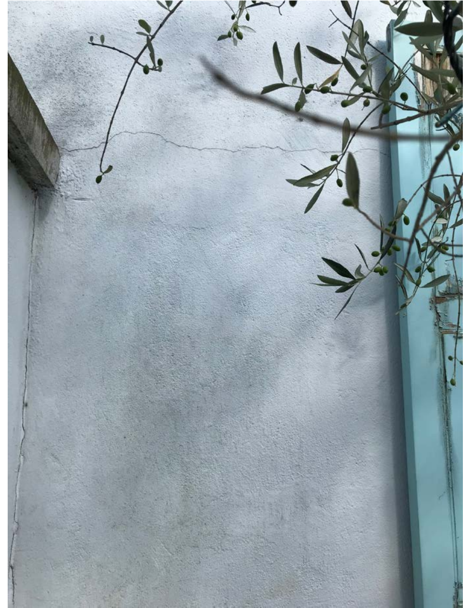
14 - Cracks to render to be made good
