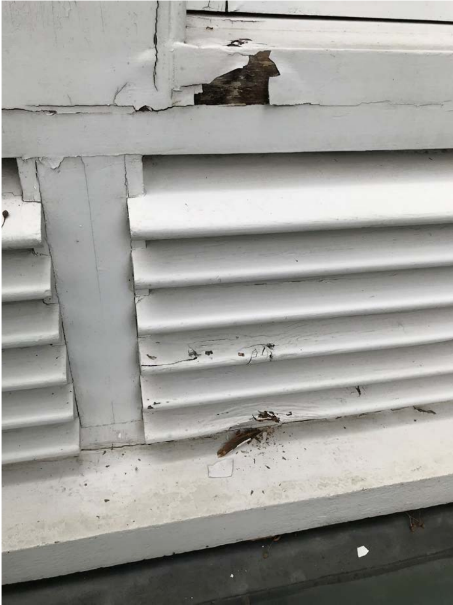
19 - Timber louvres to be replaced
