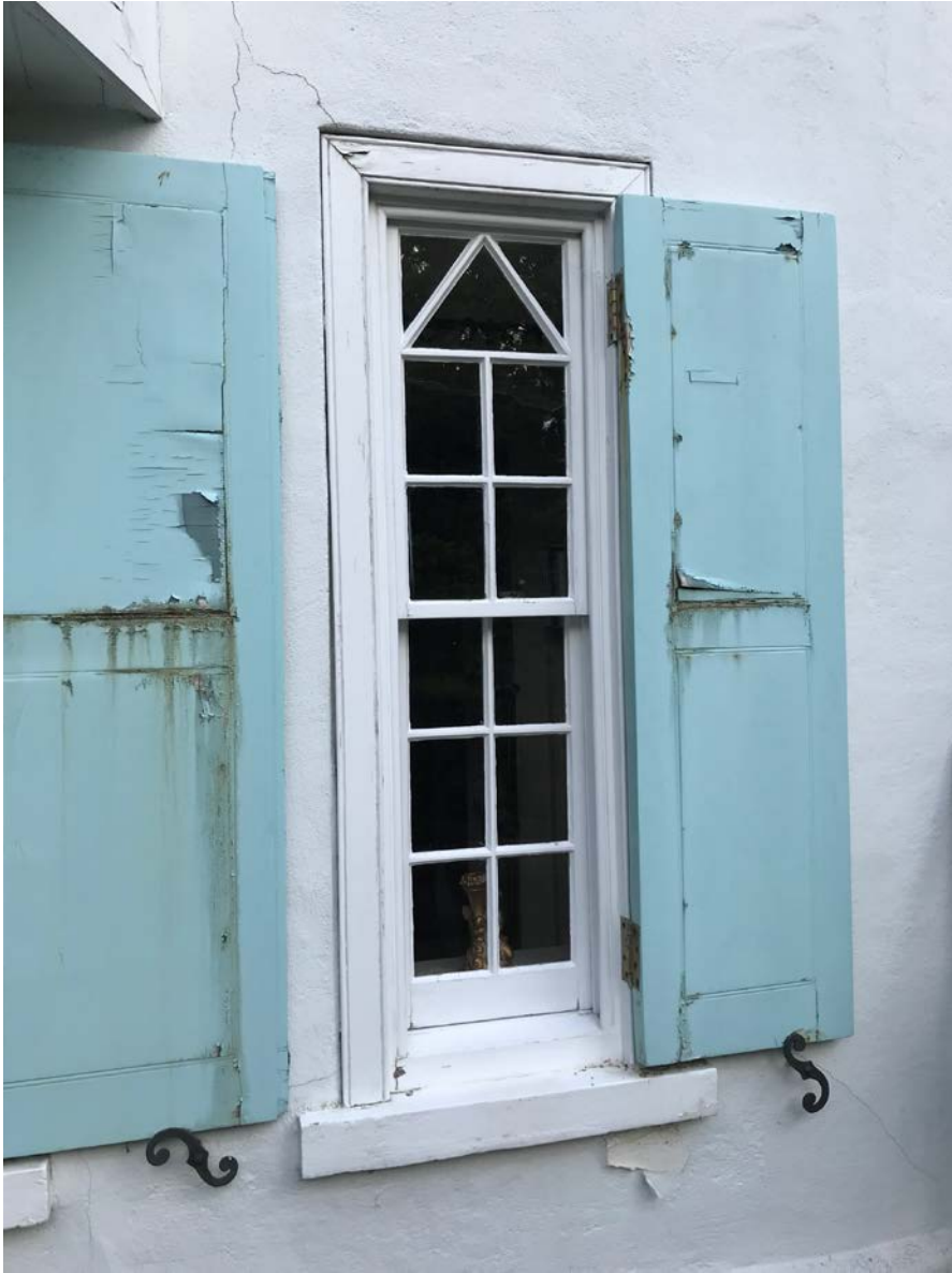
5 - Shutters to be replaced
