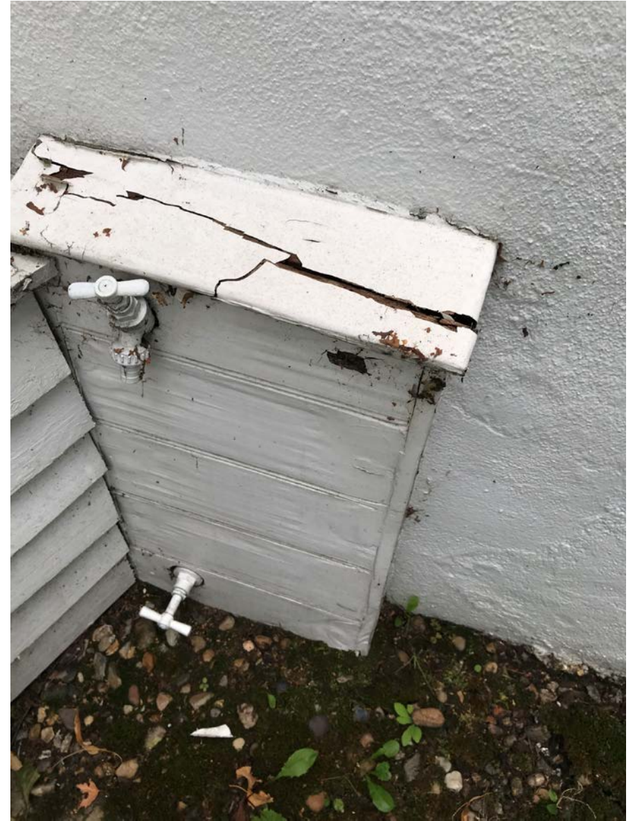
20 - Timber hosepipe enclosure to be replaced
