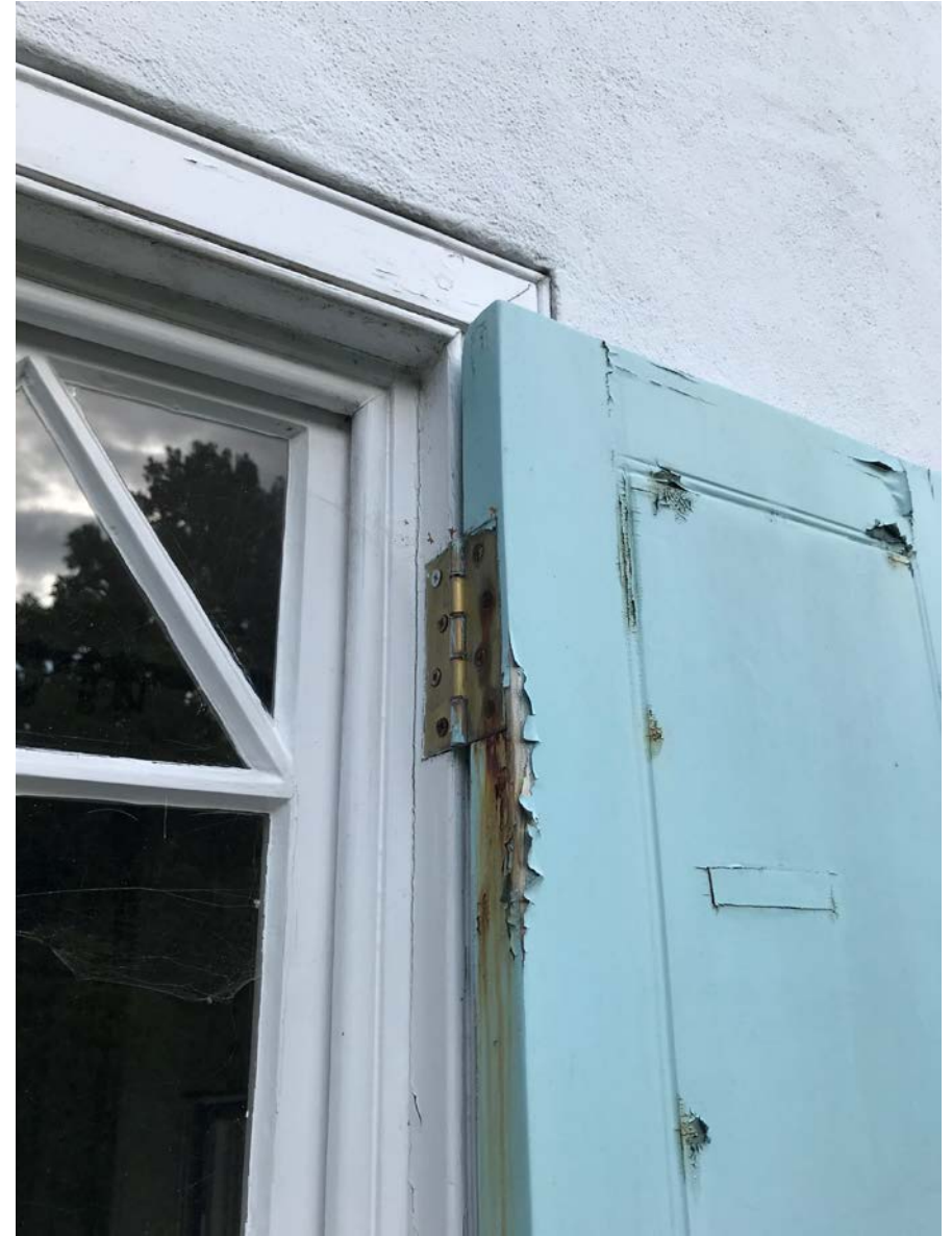
6 - Shutters to be replaced
