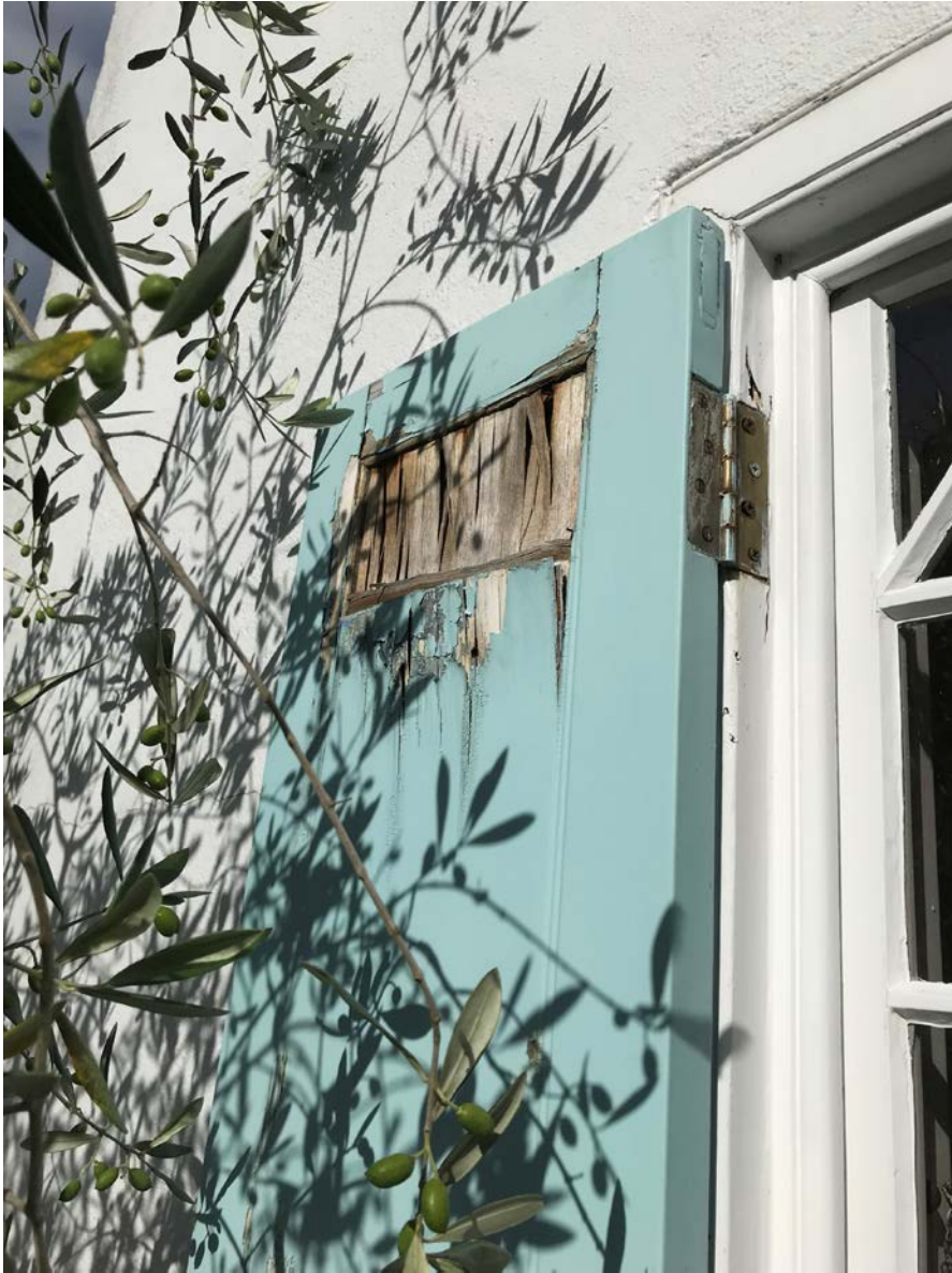
7 - Shutters to be replaced
