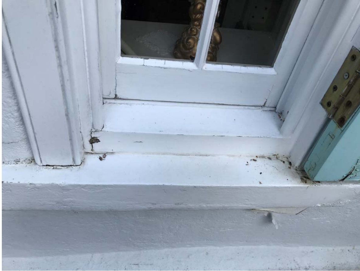
15 - Window sills to be repaired and decorated
