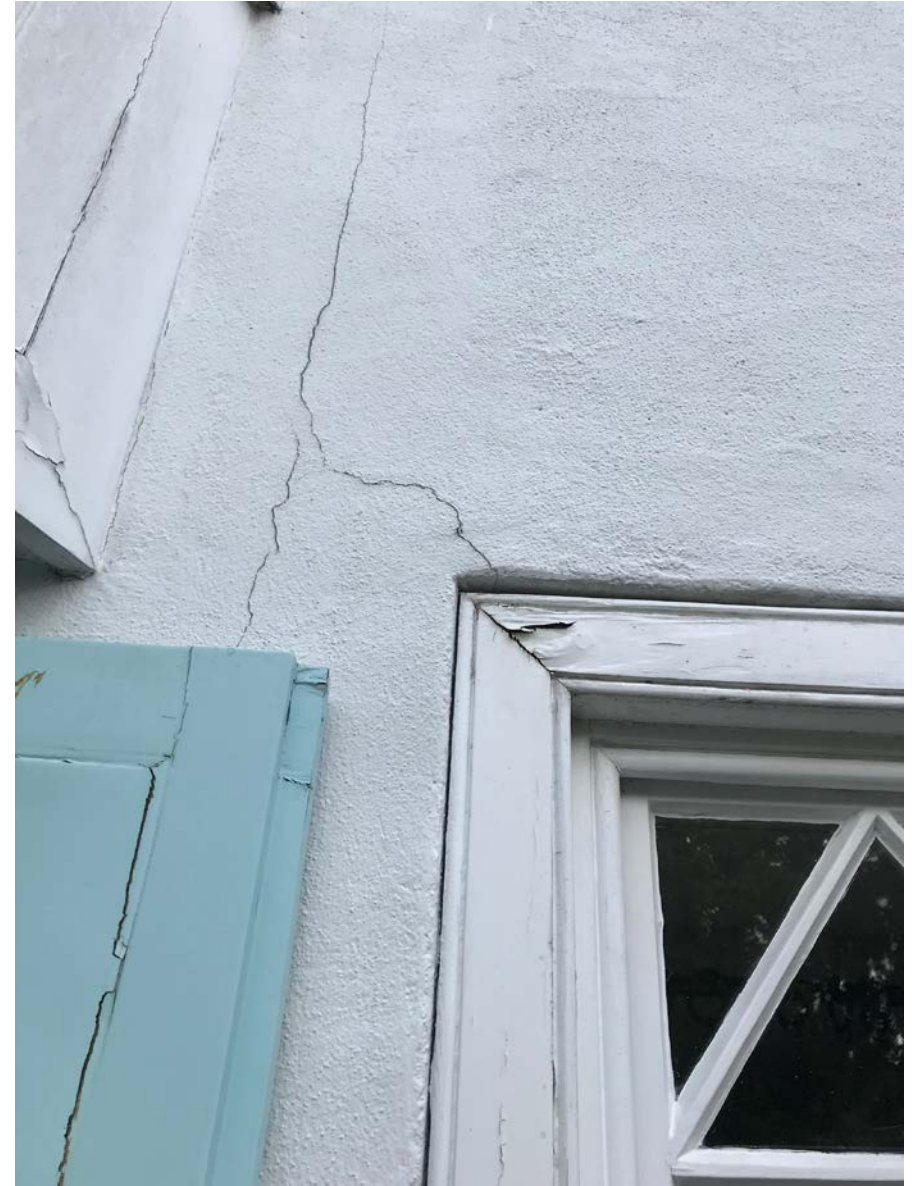
12 - Cracks to render to be made good
