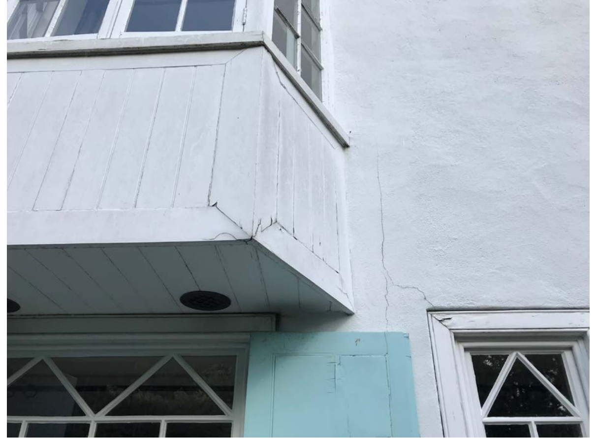
10 - Timber panelling to bay to be replaced - cracks to render to be made good
