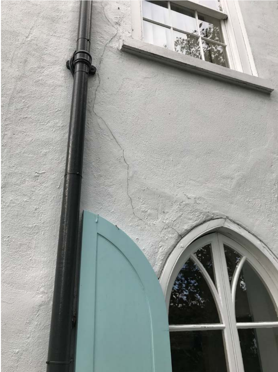
13 - Cracks to render to be made good
