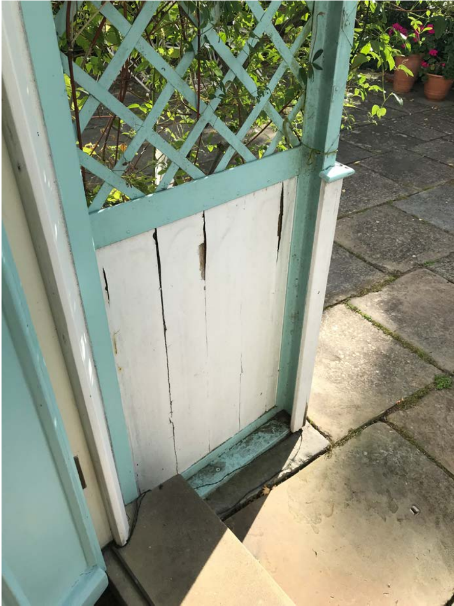
21 - Timber panelling to door entrance to be replaced
