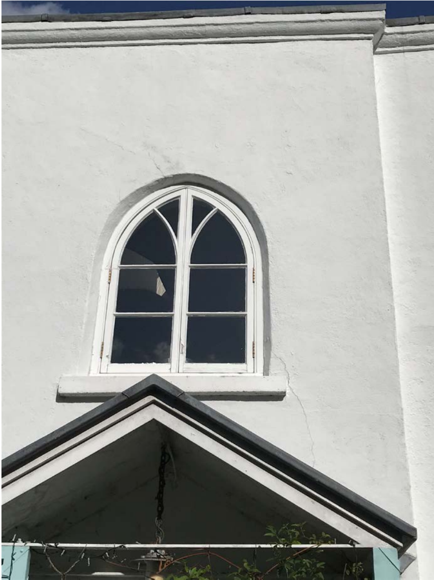
11 - Cracks to render to be made good
