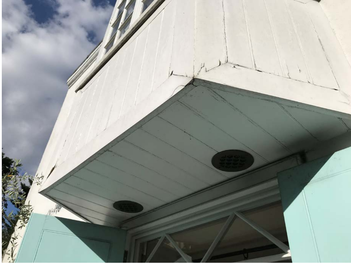
9 - Timber panelling to bay to be replaced
