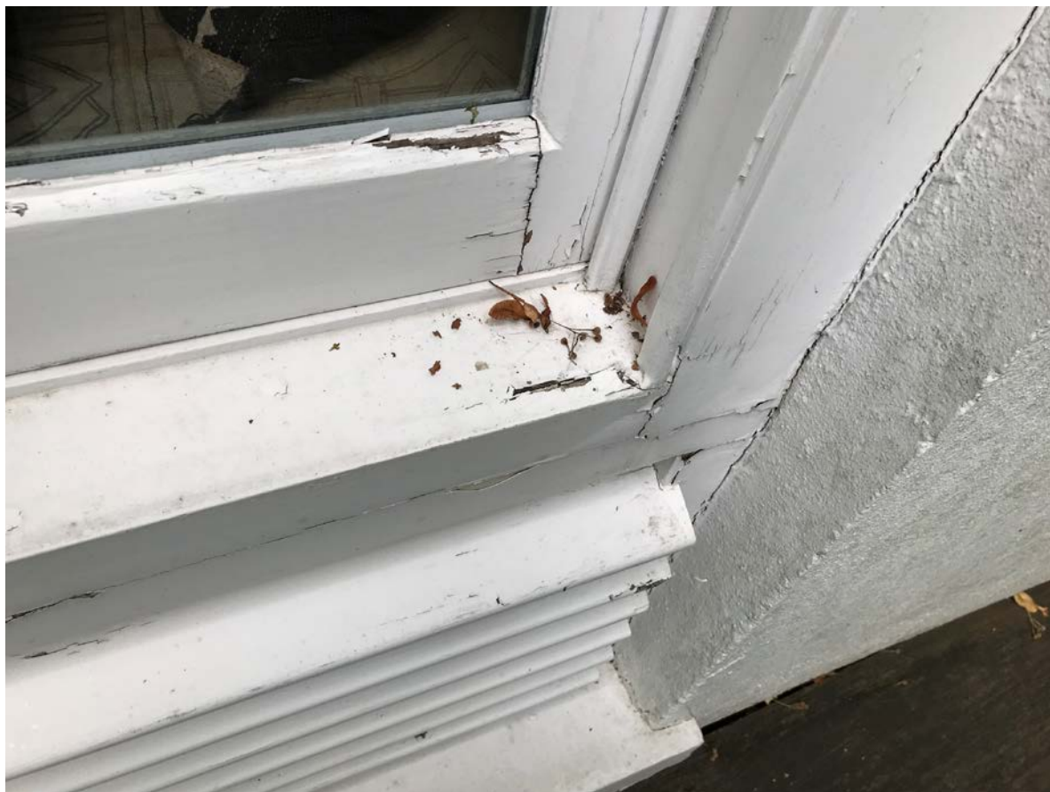
17 - Window sills to be repaired and decorated
