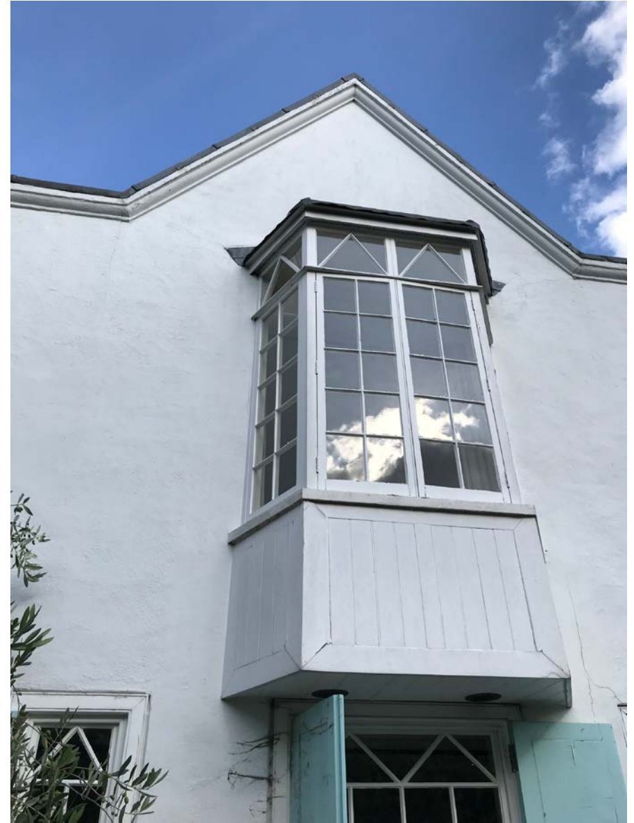
8 - Timber panelling to bay to be replaced
