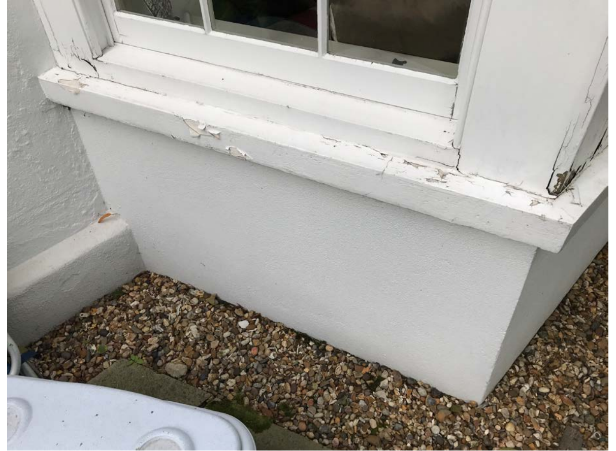
16 - Window sills to be repaired and decorated
