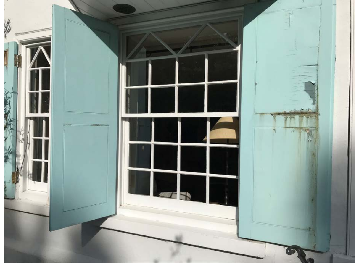
4 - Shutters to be replaced
