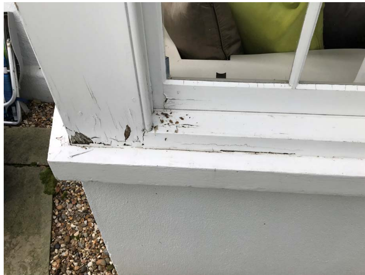
18 - Window sills to be repaired and decorated
