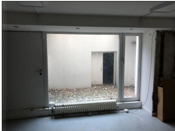
Window & Door to be Replaced
