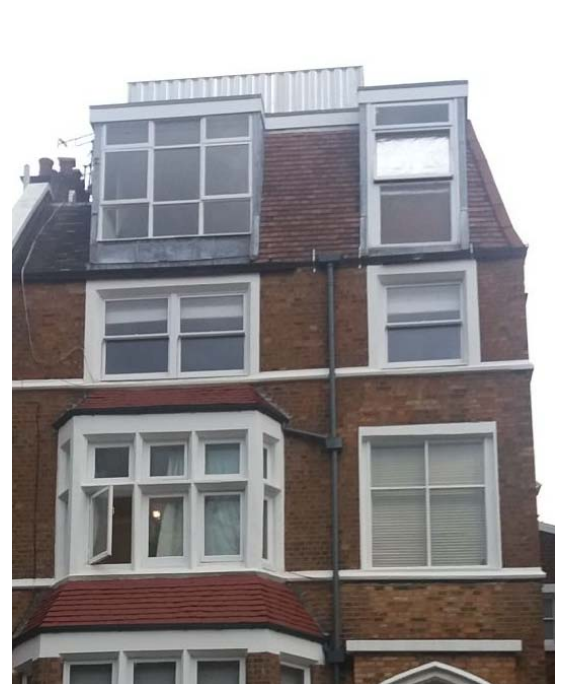
Existing single glazed timber framed dormer windows
