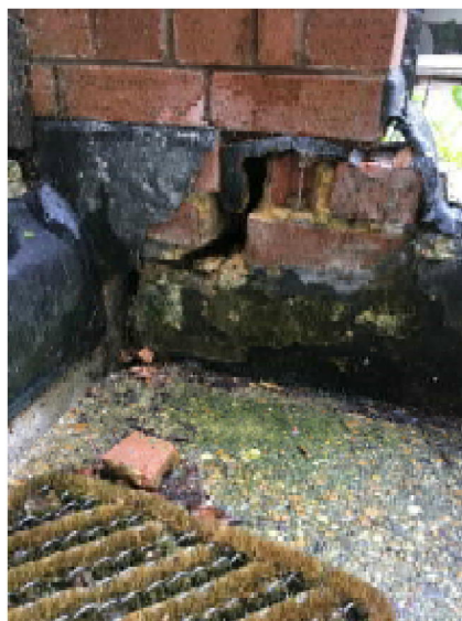
Top of staircase
