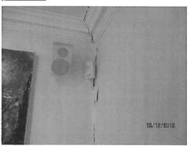
This photograph shows tapering cracking at the junction between the right hand flank wall of the lounge extension and the rear wall of the main house.
