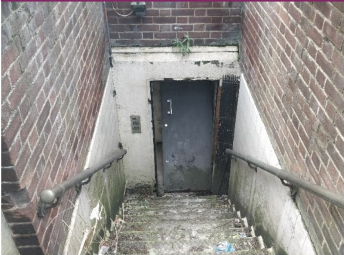
3. Stairwell down to former WC (prior to conversion) (2018)
