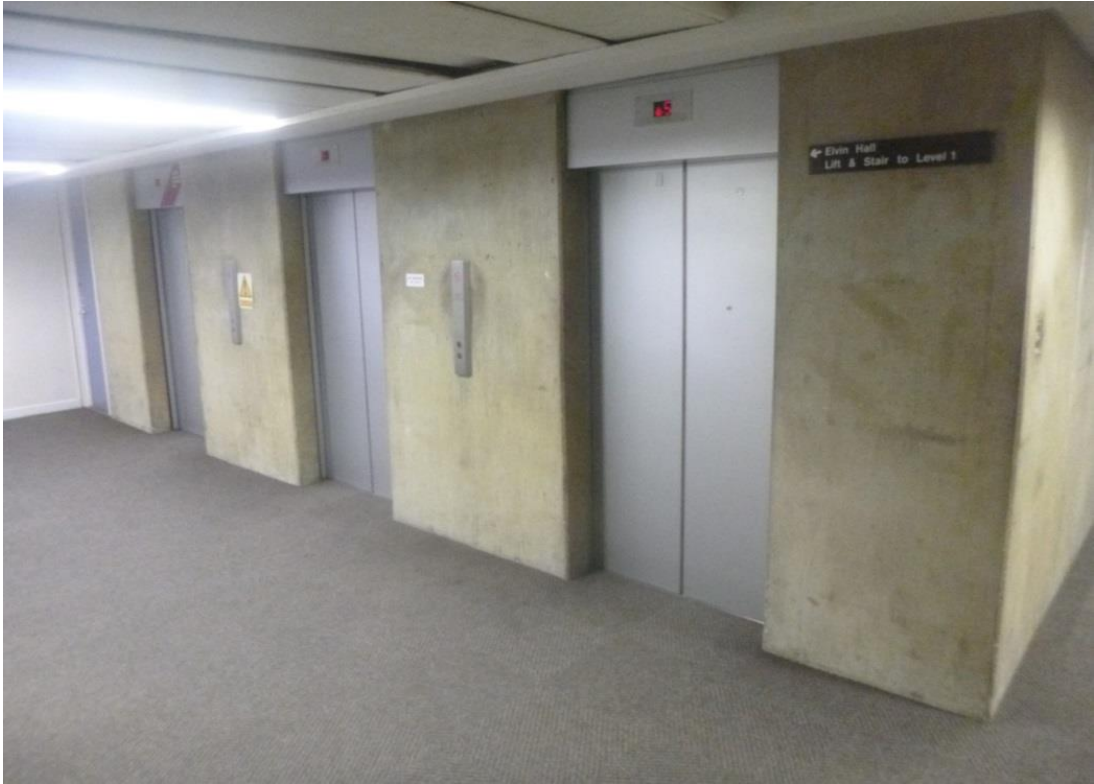
Fig. 19—High-quality concrete wall finishes in lift lobby of Core B, Level 2
