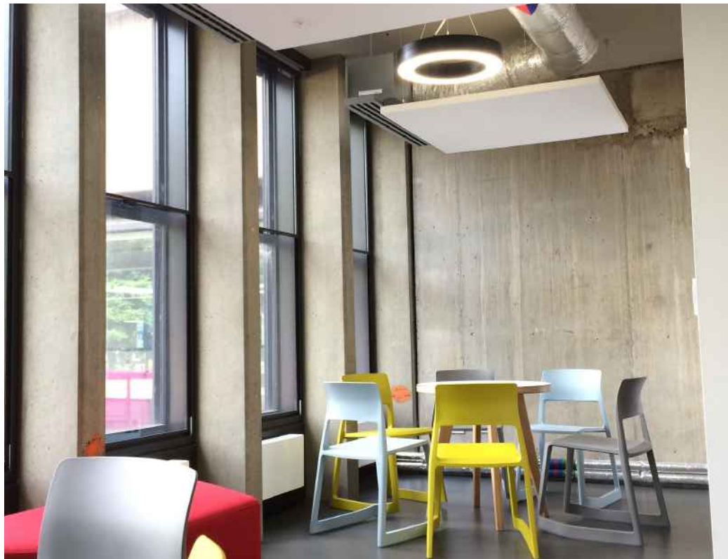
Breakout space - exposed soffits and acoustic rafts - new secondary glazing to existing facade to Phase 1, Level 4
