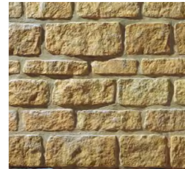
Stone Clad Retaining Wall
