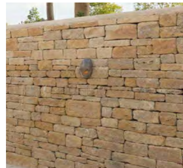
Wall Mounted Lighting
