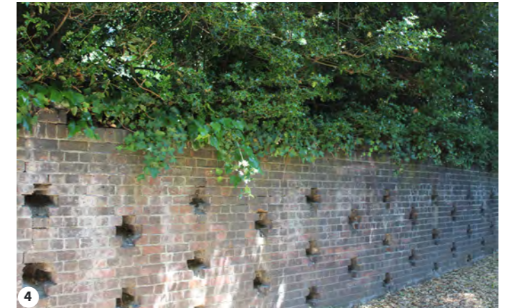
4 EXISTING RETAINING WALL TO SOUTH ACCESS ROAD
