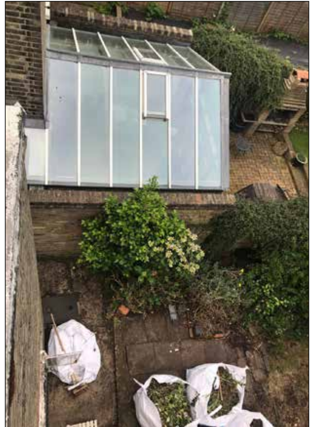
Fig 8. Existing view of No.7's full width extension from upper floor flat - 2019.
