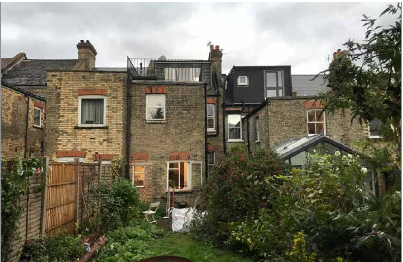
Fig 5. Existing rear elevation - November 2019.
