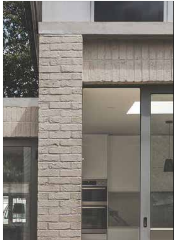
Fig 18. Example of concrete coping with brick piers and lintel for rear elevation.
