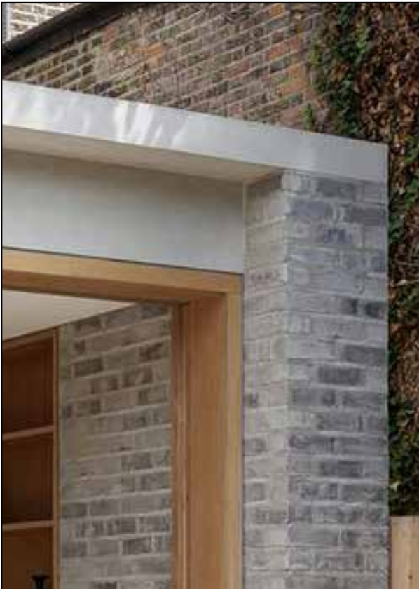
Fig 17. Example of brick and concrete for rear elevation.
