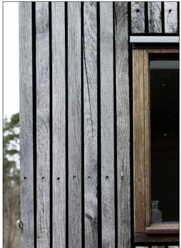
Fig 20. Example of timber slatted rainscreen for garden outbuilding,
