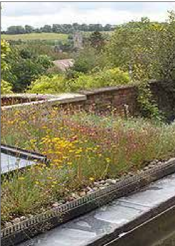
Fig 19. Example of living sedum roof.
