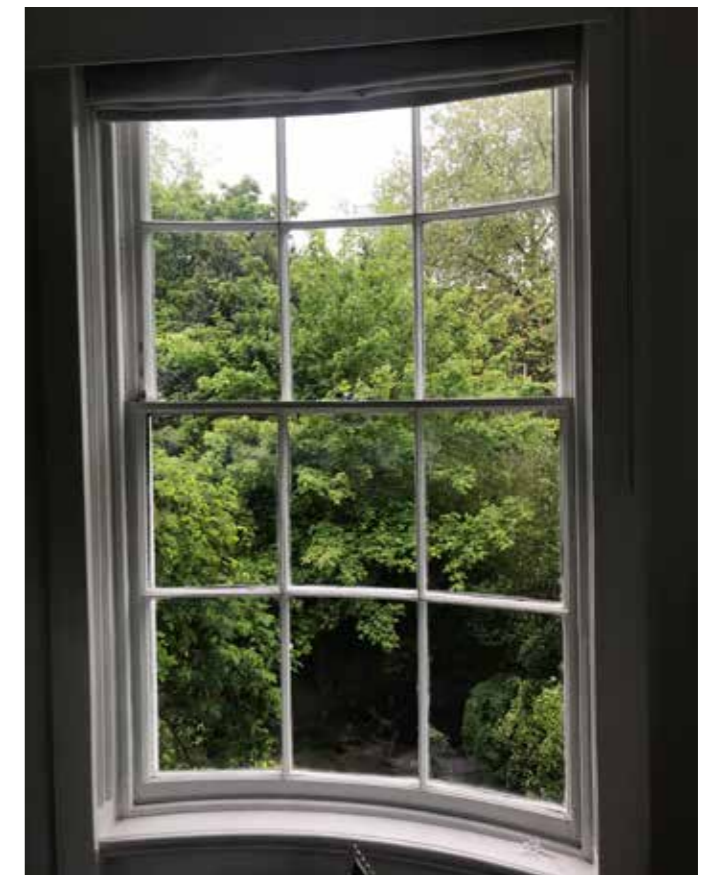
Figure 5.2 The curved windows to Bedroom 1
