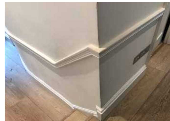
Figure 5.1 Curved wall to first floor bathroom (left)
