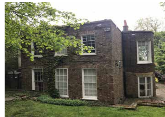
Figure 4.2 Rear facade of the 1973 extension and earlier bay
