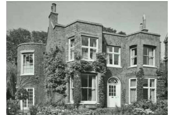
Figure 3.5 Photograph of Site 1951
