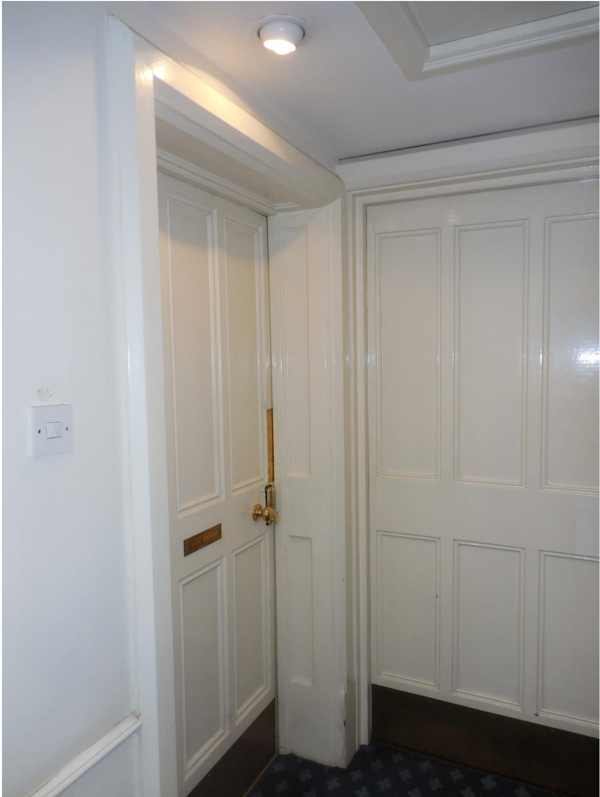
FIG.6 – DROPPED CEILING IN LOBBY 4 TO BE REMOVED AND EXISTING CONCEALED VAULTED CEILING TO BE RE-INSTATED
