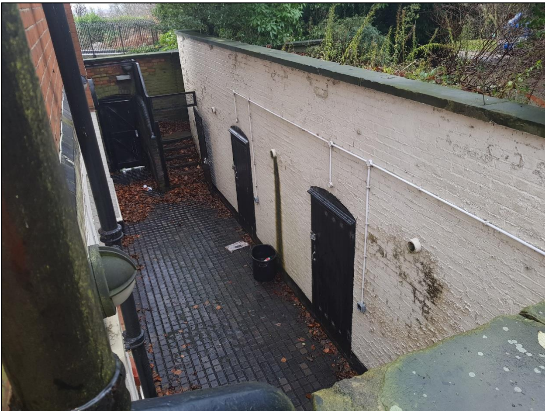
h) Basement rooms viewed from ground level
