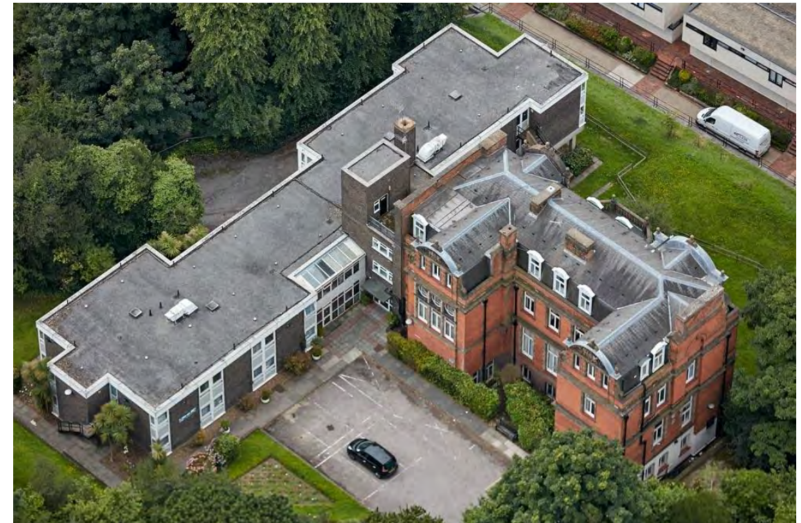
Figure 12: The Edwardian building is basement and two storeys with an additional floor within the mansard roof extension. The house is 'C' shaped in plan aligned roughly along the north-south axis with the two wings extending to the east. Since the site on which the house is placed is sloping down towards the west side, the ground floor is accessed only from the west side.
