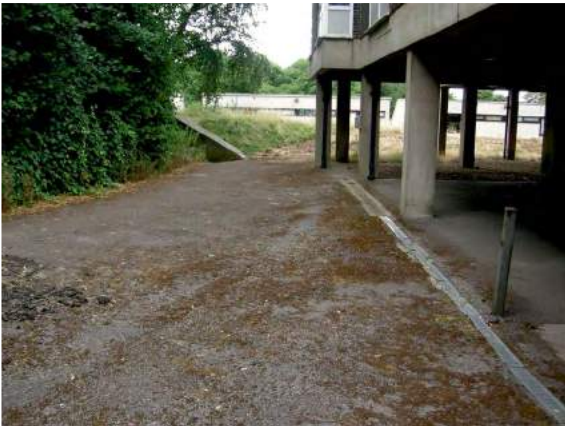
Fig 17 View of open area below ground floor of modern extension building (MOLA photograph, 17/07/2018)
