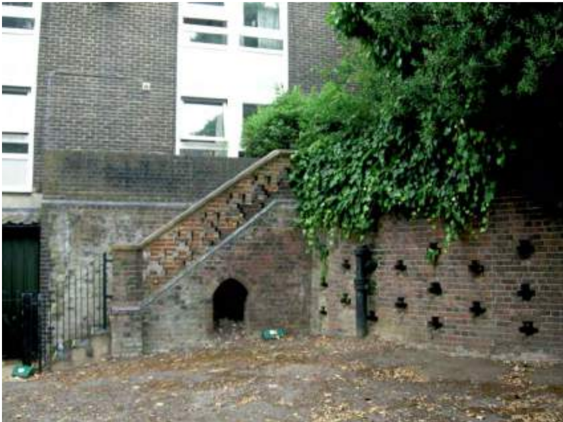
Fig 15 View of retaining wall, facing north-west (MOLA photograph, 17/07/2018)
