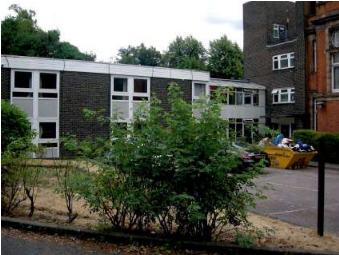
Fig 16 View of modern extension building abutting Branch Hill House, facing south-west (MOLA photograph, 17/07/2018)
