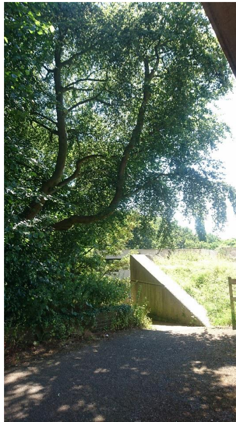
Photo 3 showing ungainly form of T14 to be removed
