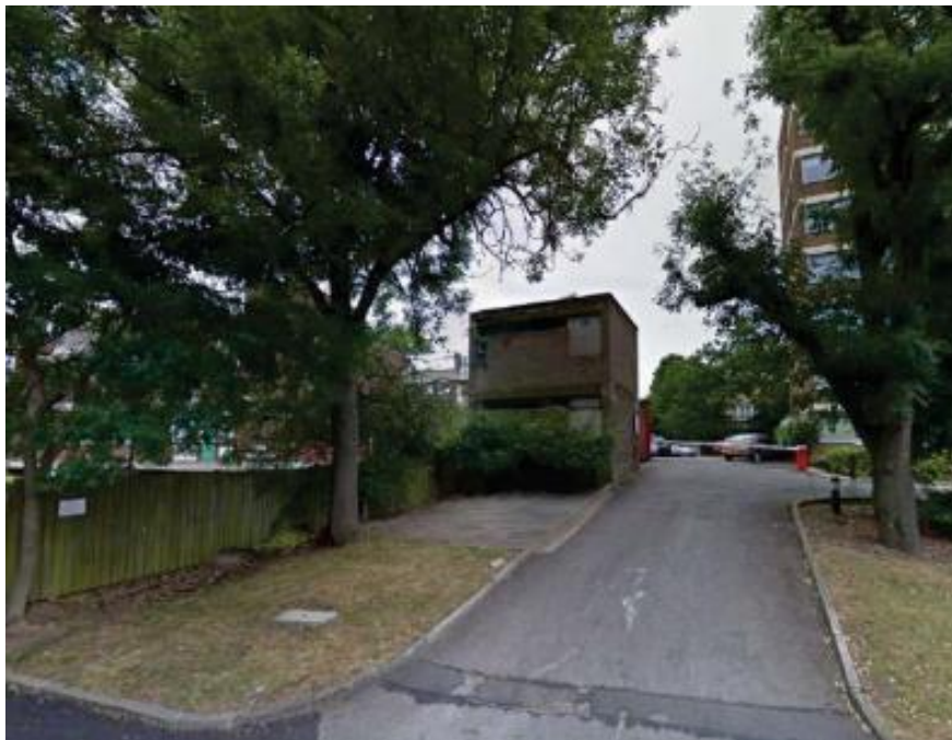
Above: View of existing vacant porters lodge to the north west of the main block
