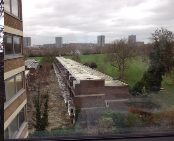
Above: View of Kingsland from the upper floor flat in the southern block of Barrie House
