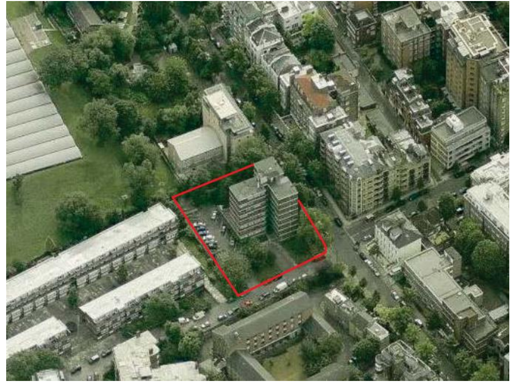
Above: Ariel view of Barrie House looking east
